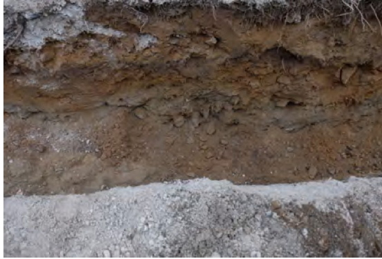
Figure 4 Dug pit for water line
