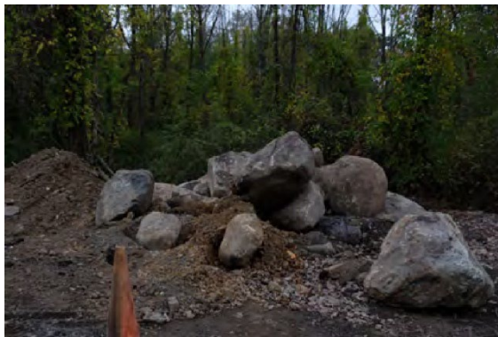
Figure 5 Large rocks dug up during construction
