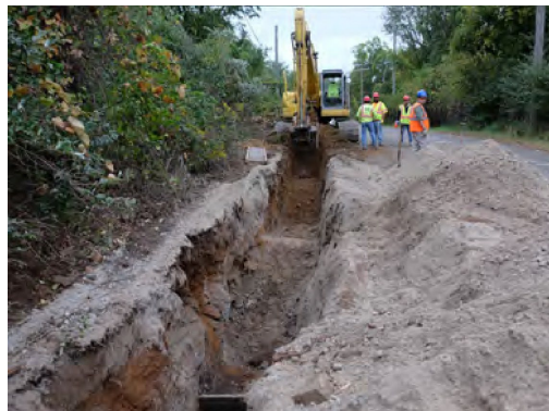
Figure 3 Water line construction
