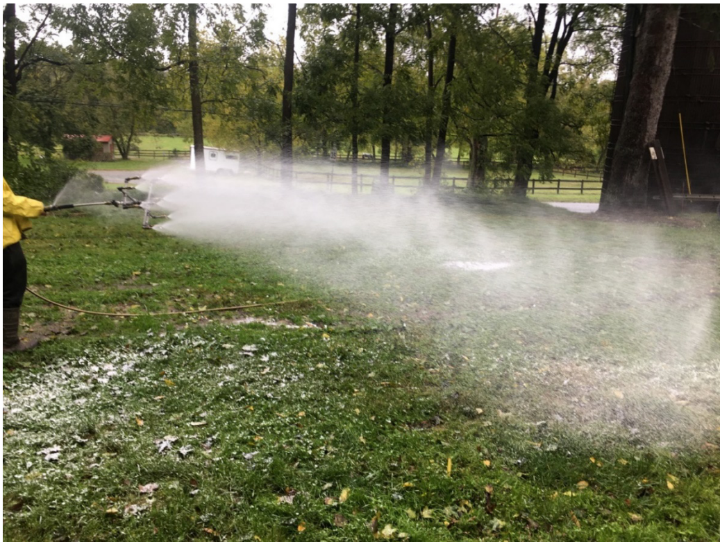
Photo 3. Pressure Washer with Foam Cannon (9 mist nozzles)
