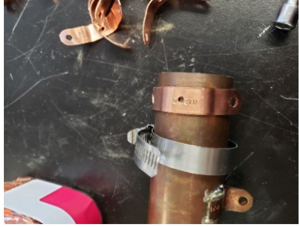
Figure S3.6. The Strap Was Placed on the Same Scrape Pipe.
