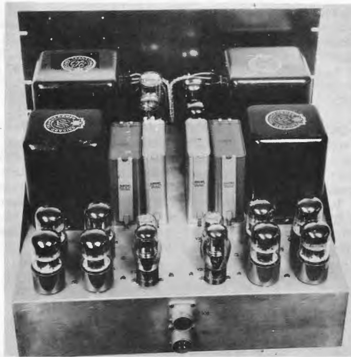
Fig. 16 - Power supply 1 and 2
