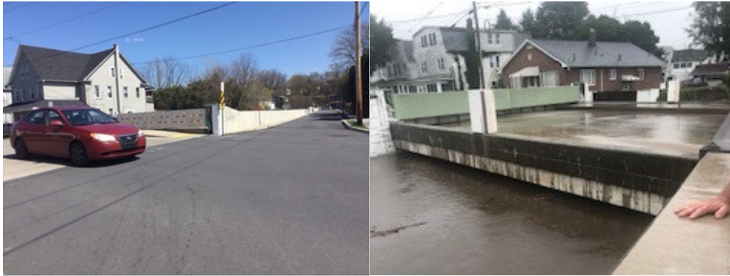
Figure 11. Solomon Creek Bridge 303
