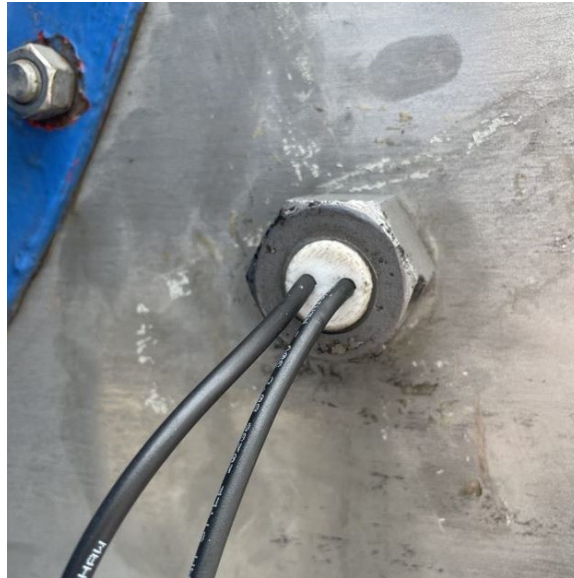
Figure 3.4. Airtight Connection
