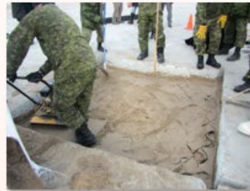
Sand-filled geocell backfill
