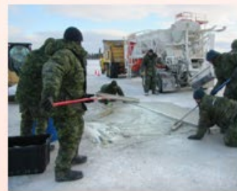
Rapid-setting concrete cap placement
