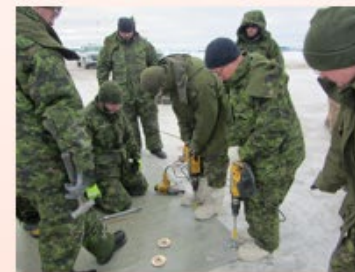
Fiber reinforced polymer (FRP) matting installation
