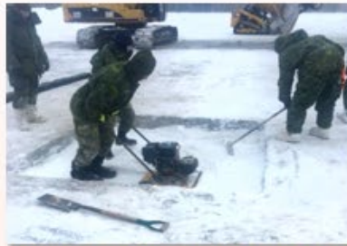
Snow-water slurry backfill
