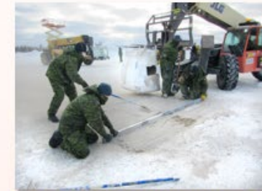
Rapid-setting flowable fill backfill
