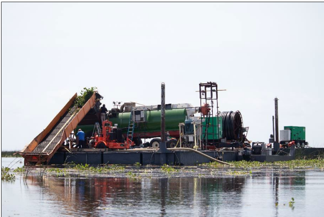
Figure 2. Floating barge containing a plant elevator, macerator press (juicer), generators, and a hydraulic pump.
