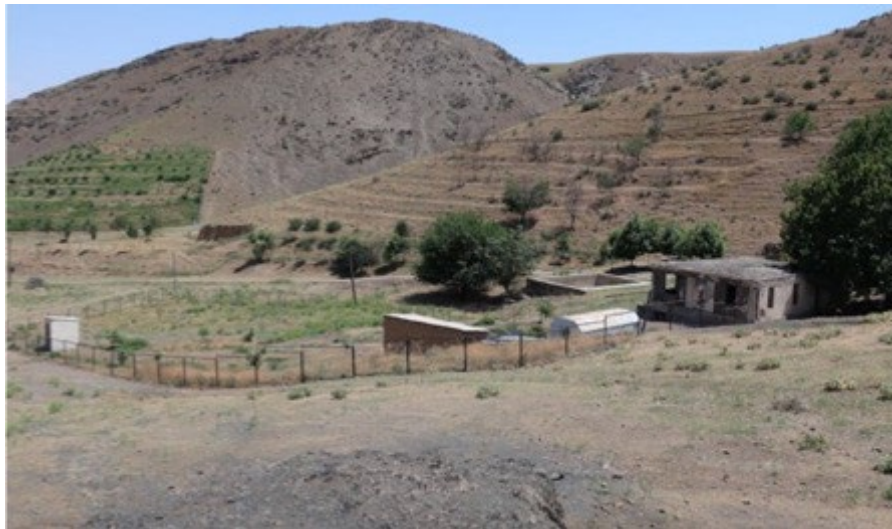
Figure 6. View of the station from the hillside above in 2018. The tunnel extends into the hillside.
