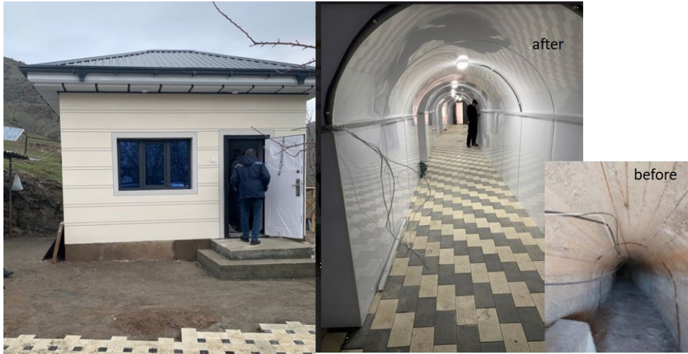
Figure 14. Photo of newly constructed station building (left) and tunnel (right) showing improvement (before tunnel photo shown for comparison).
