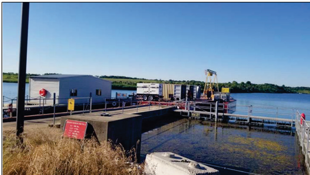
Figure 24. Equipment on the floating pier system after setup.
