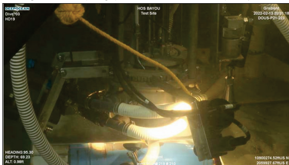
Figure 21. Subsea photographs of the Underwater Cut and Capture System.
