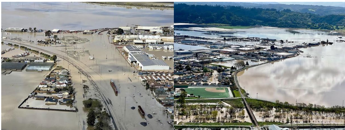
Figure 4. Aerial photos of the City of Pajaro flooding. Source: Jimenez (2023).
