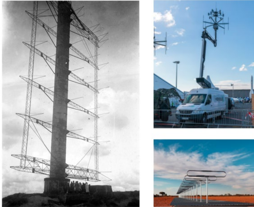
(Left) Antenna of Klein Heidelberg. The first application of a passive radar was in the 1940s. Source: [11]. (Right) Antennas of modern passive radars. At the top right panel, Hensoldt's TwinVis passive radar system for air defense is presented, while the bottom right panel shows the Silentium Defense Maverick S-series air and space search radar.
