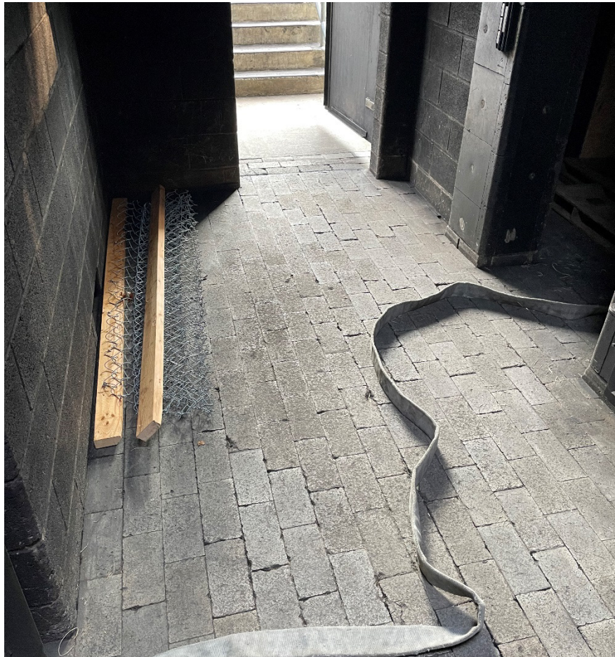
Figure 9. Ceiling collapse prop
