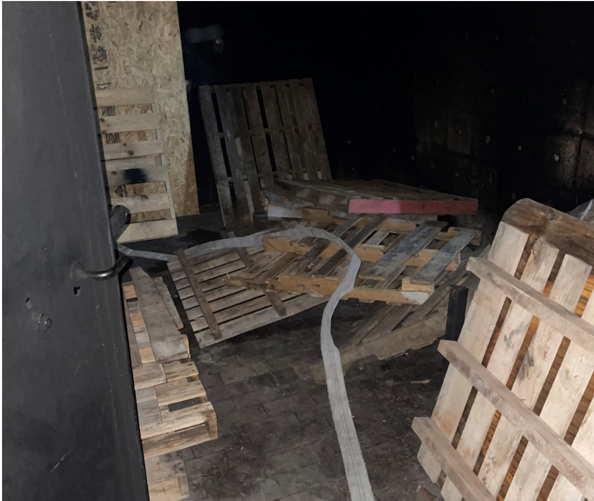
Figure 11. Pallet debris with hoseline
