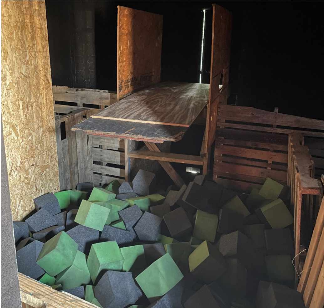
Figure 3. Floor collapse prop
