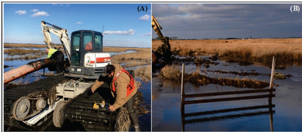
Figure 5. (A) Pontoon excavator relocation equipment and (B) witness boards for tracking TLP elevations. (Image reproduced with permission from McCullough et al. 2021.)
