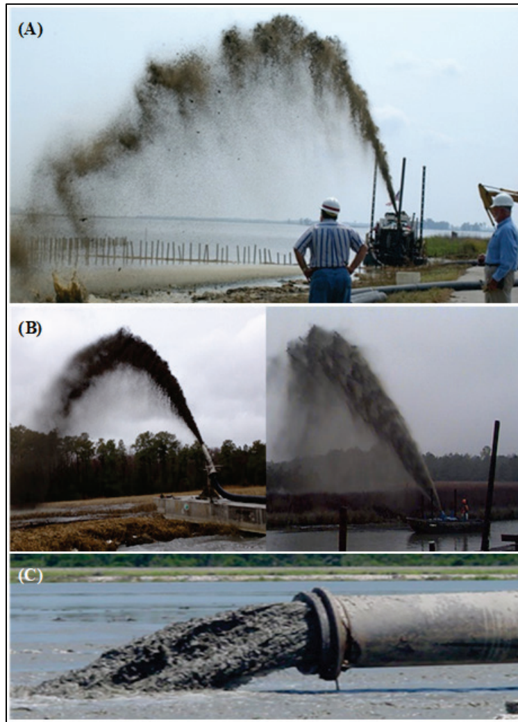
Figure 2. Standard methods of thin layer placement (TLP): (A) direct spray from a dredge; (B) spray from a pontoon barge or small boat (fed by pipelines); (C) traditional pipeline application. (Image reproduced from Piercy et al., in preparation. Public domain.) 2
