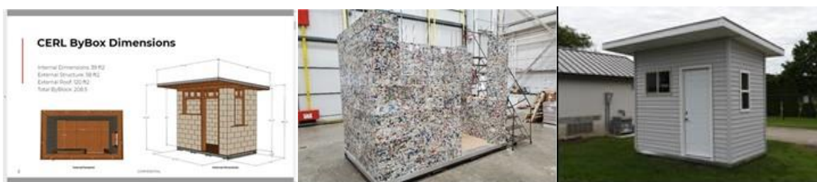
Figure ES-6 Demonstration project at ERDC-CERL - a storage shed designed and built with mixed plastic waste ByBlocks
