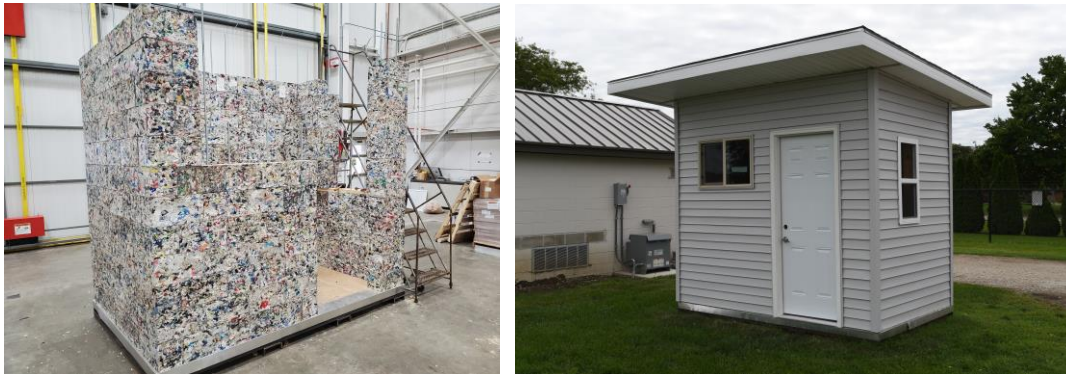
Figure 28. Photo of storage shed under construction and completed at ERDC-CERL
