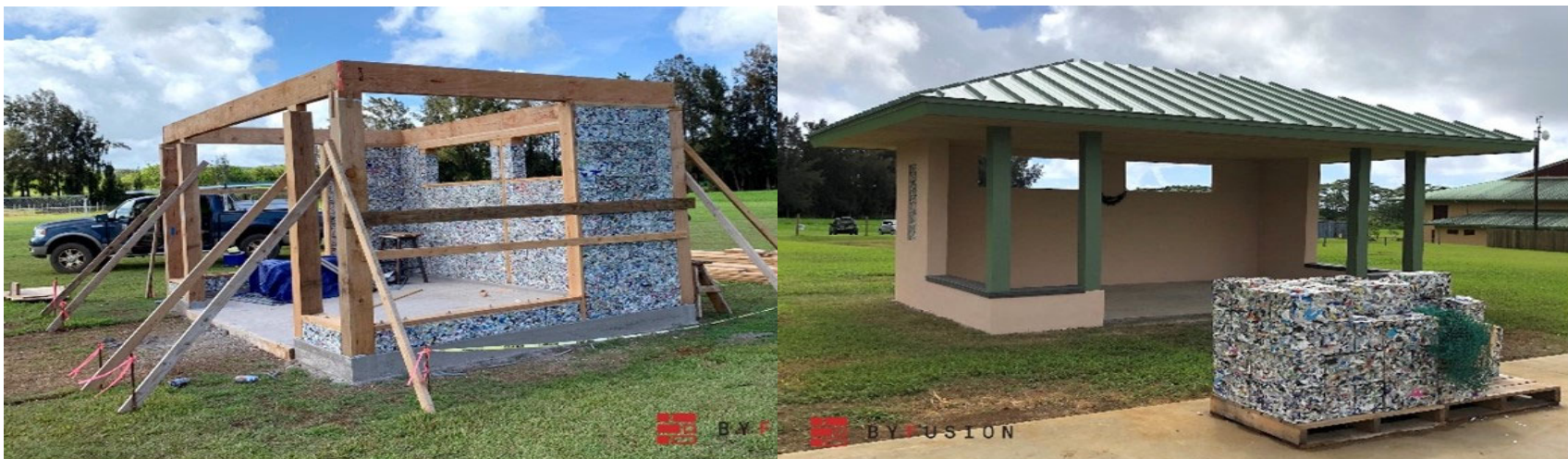
ByBlock Pavilion Installed in Kauai, HI
