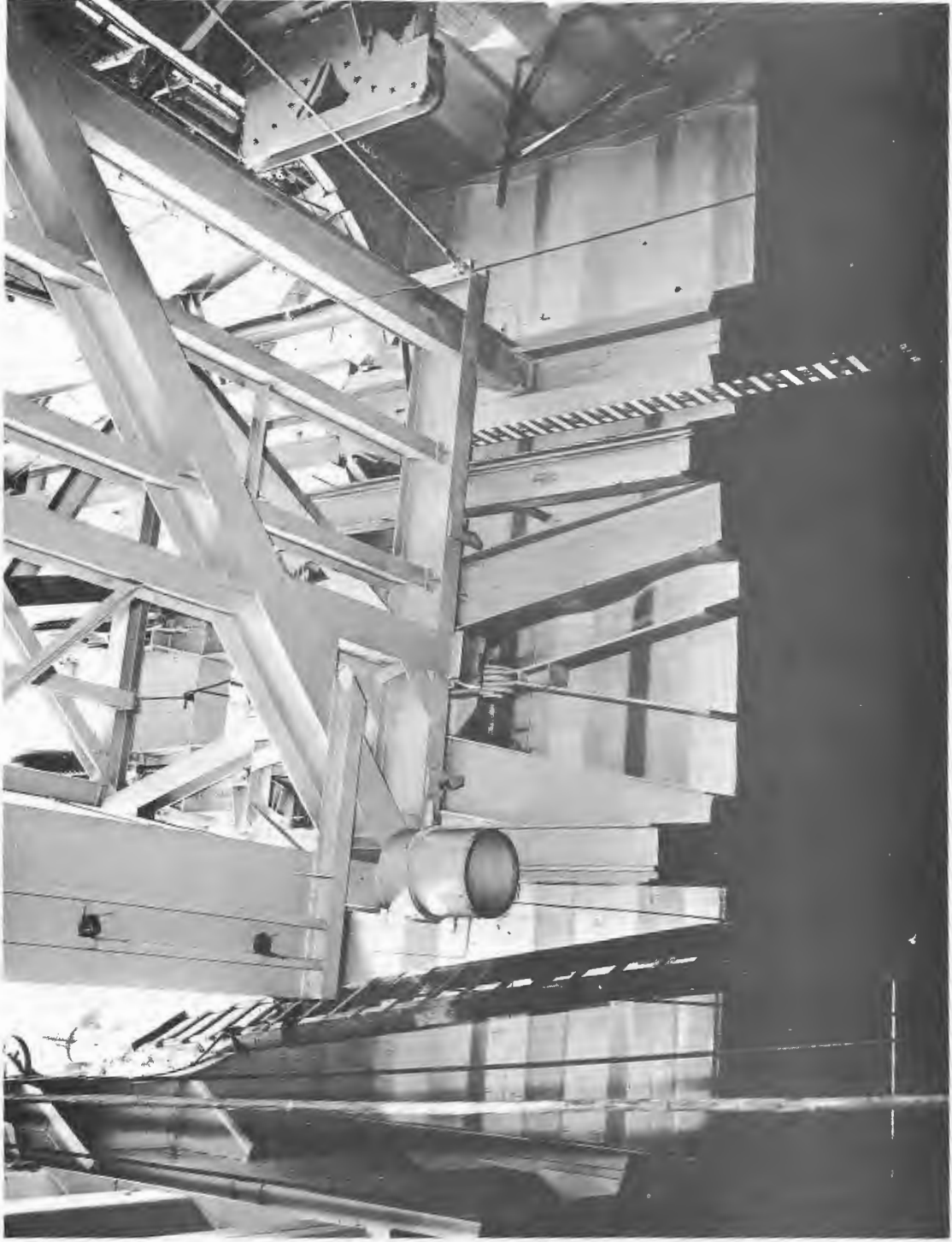
Figure 76 - Array support structure in raised position viewed from below, looking aft
