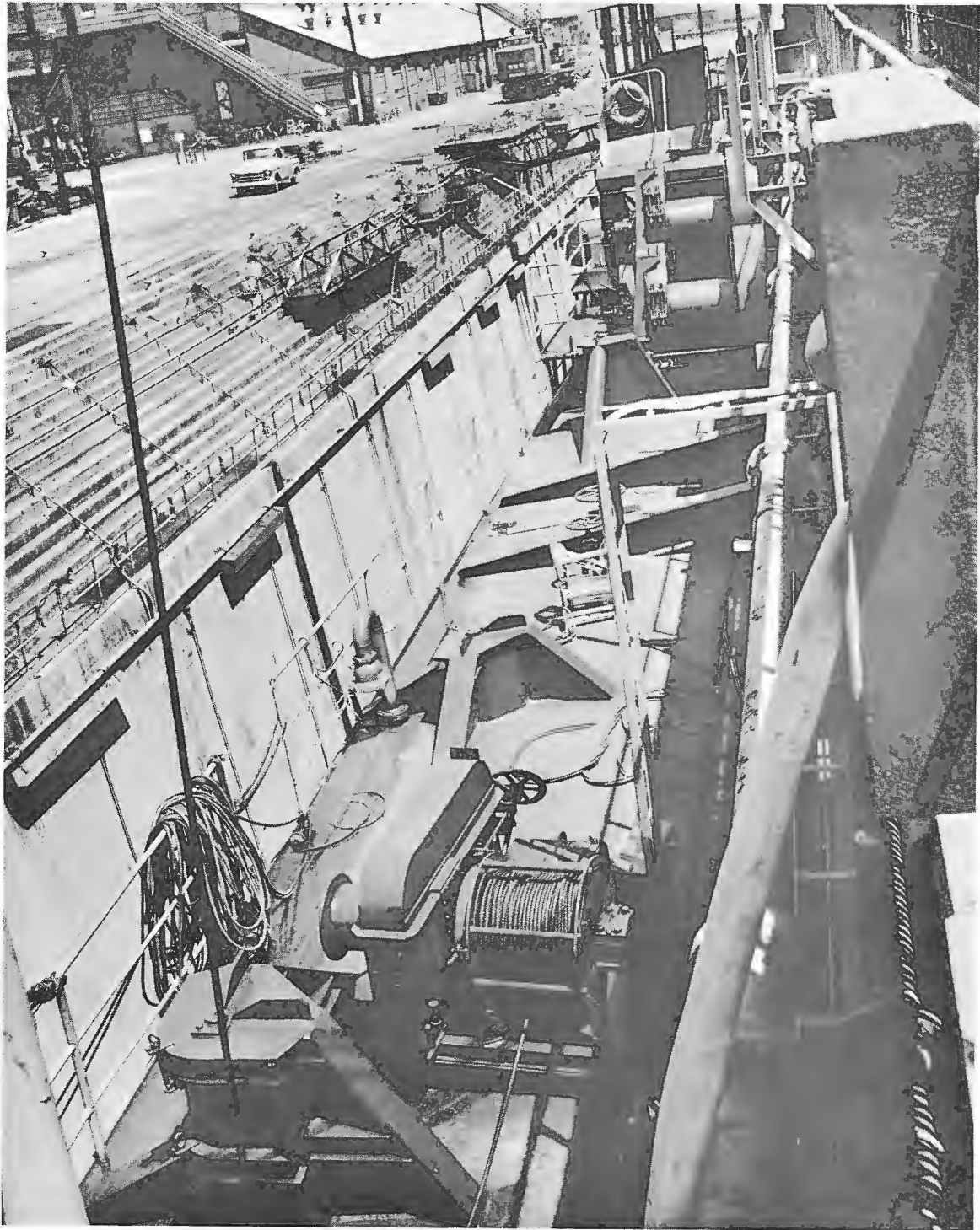
Figure 17 - Deck layout, port side, approximately midship to the deck house
