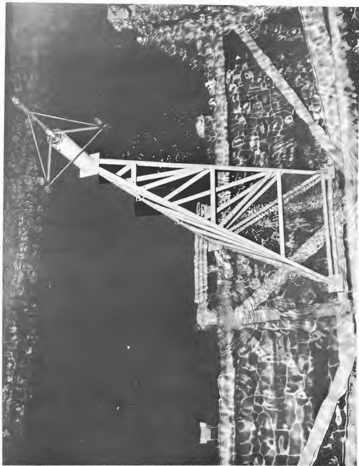
Figure 81 - Position determining system hydrophone array showing array structure partially submerged
