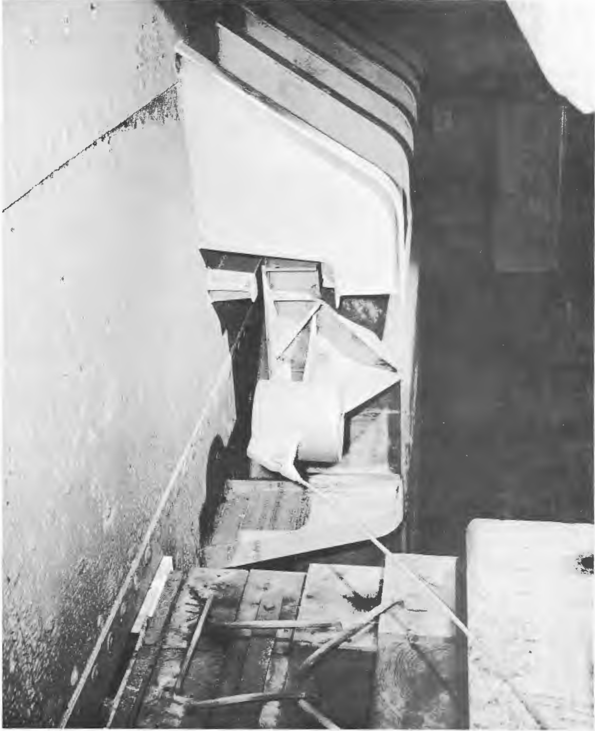
Figure 26 - Wire rope termination and locking pin sleeve on forward part of well door
