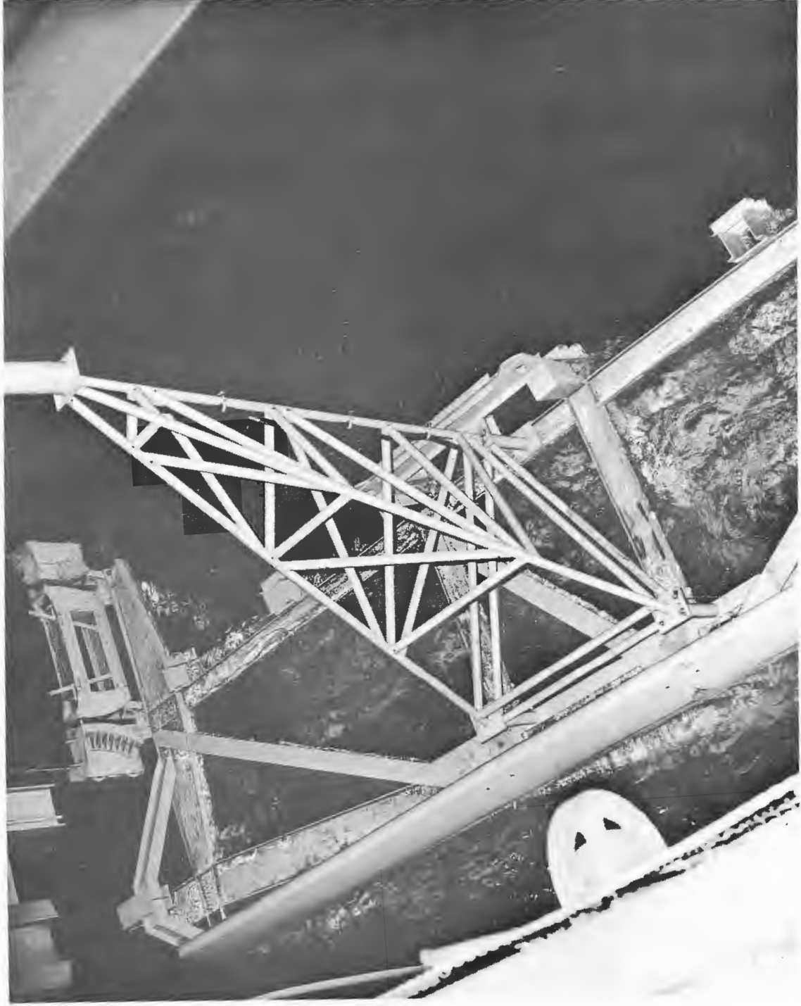
Figure 80 - Array structure with top beam wash showing PDS and wire rope roller path guide
