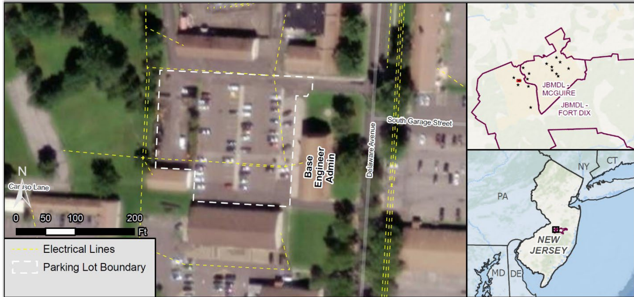
Figure 2-4k. JBMDL 787 th Civil Engineer Squadron Building 5320
