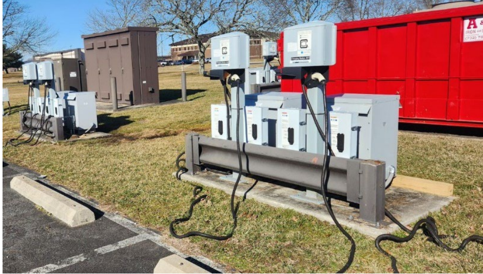
Figure 2-1b. Example Free-standing Level-2 Charger
