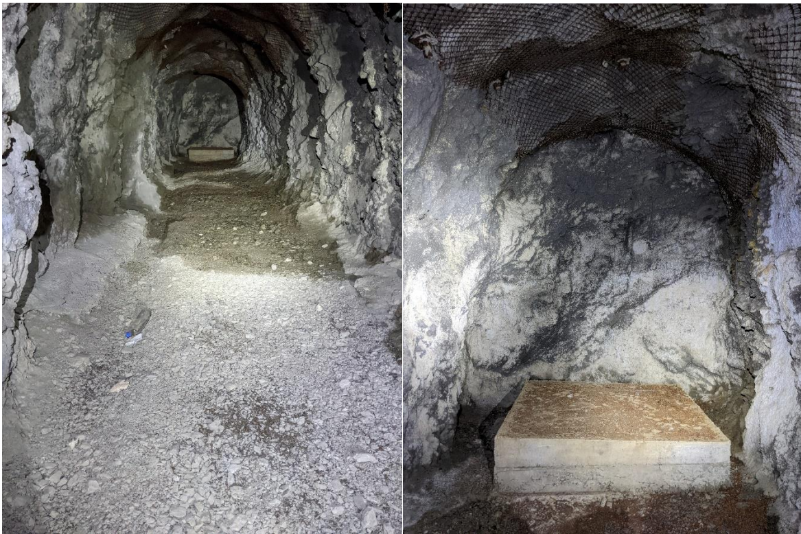
Figure 47. Left – looking down the tunnel to the pier at point 5. Right – The pier at point 5. Note the shotcrete walls and rockbolts with mesh on the ceiling.
