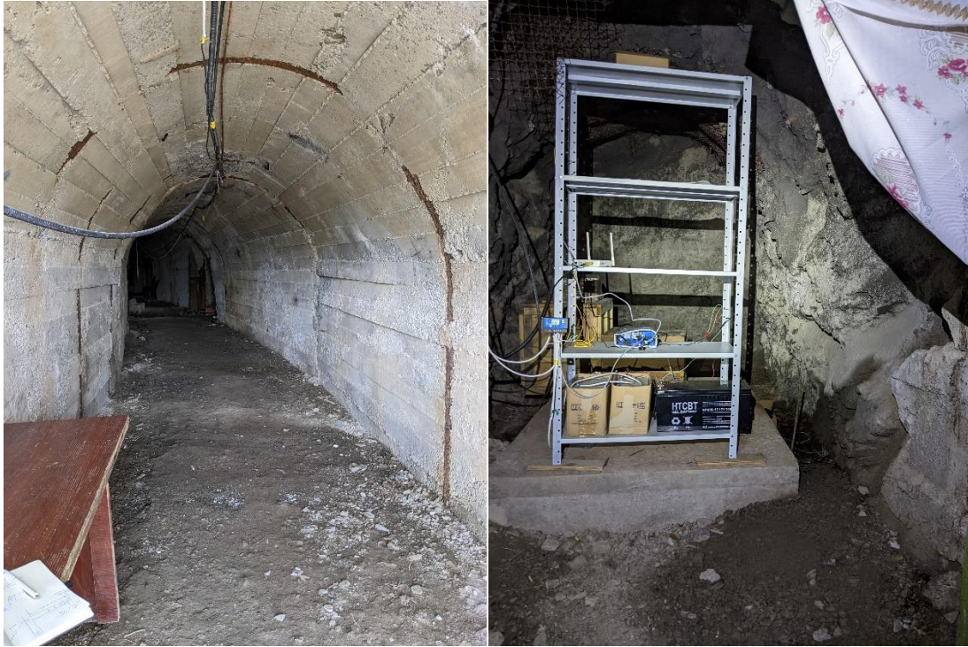
Figure 46. Left – Looking into the tunnel from near the entrance and showing formed concrete walls. Right – The current instrument rack on the pier at point 1.
