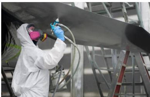
Figure 1. Spray application of a coating to an aircraft surface
