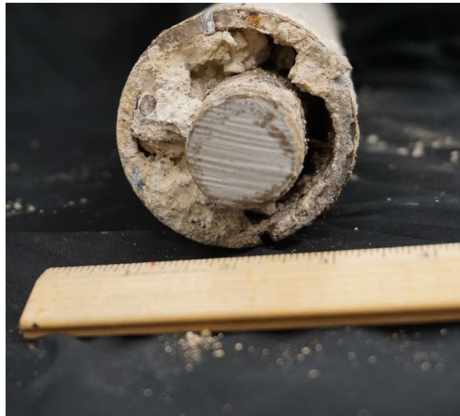
Figure 48. Core 210043-1 pipe sleeve end-on view.
