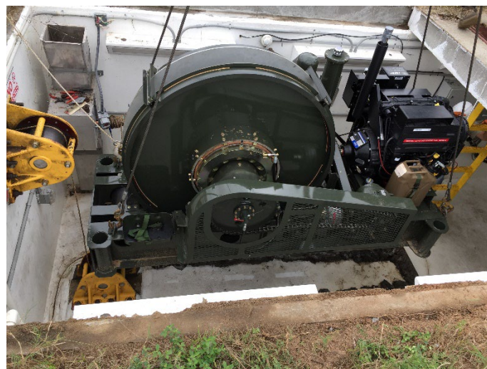
Figure 1. Barrier Arresting Kit 12 being lowered into an installation pit.
