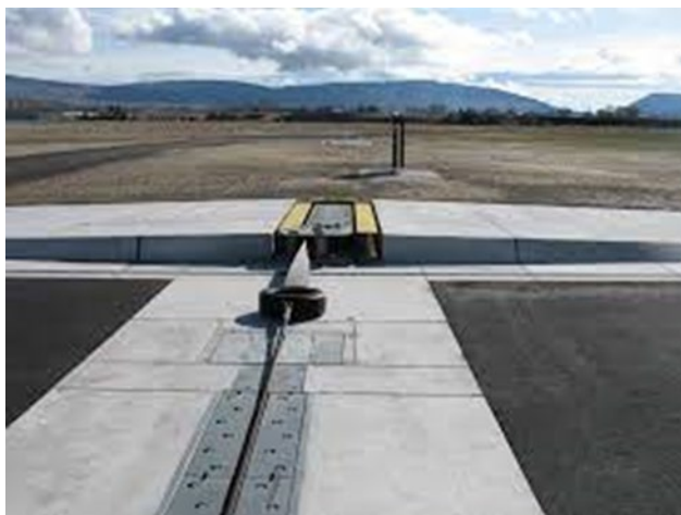
Figure 2. Permanent fairlead beam installation.
