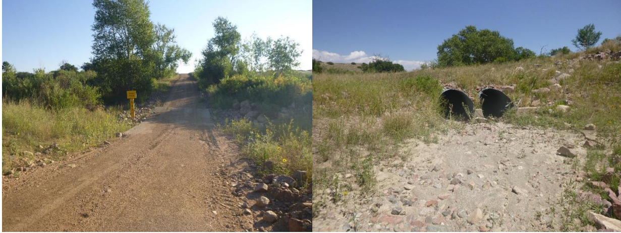
Figure 4.10: A typical improved ford LWC (FC04, left) and vented LWC (FC05, right) at Fort Carson.
