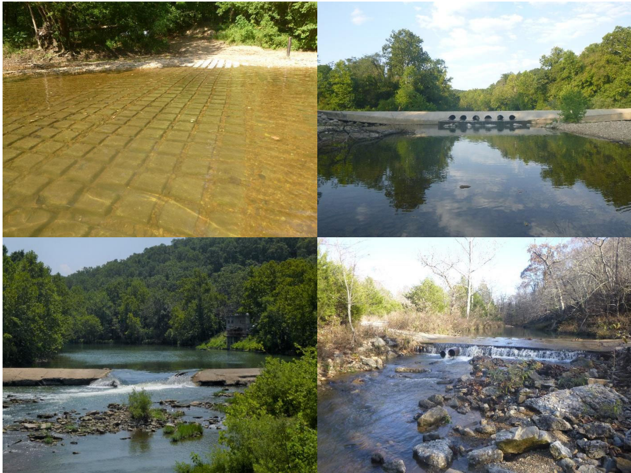
Figure 4.6: A typical improved ford LWC (FLW03, top left) and vented LWC (FLW02, top right) on Roubidoux Creek. Low head dam and potable water intake on the Big Piney River (FLW13, bottom left). Typical vented LWC (FLW04, bottom right) on Turnbull Hollow.
