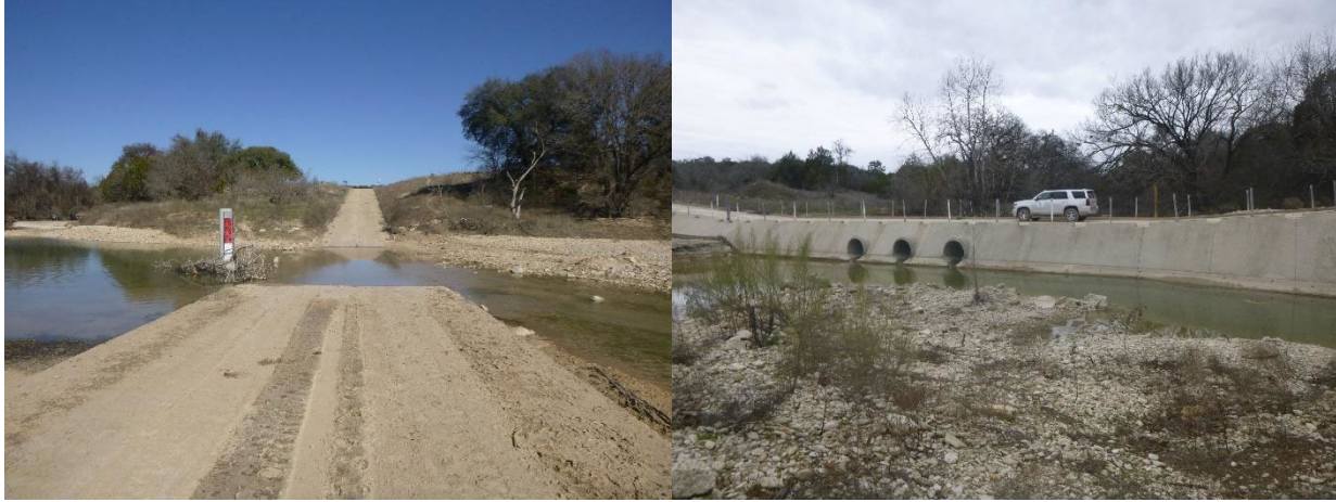
Figure 4.2: A typical improved ford LWC (FH21, left) and vented LWC (FH01, right) at Fort Hood.
