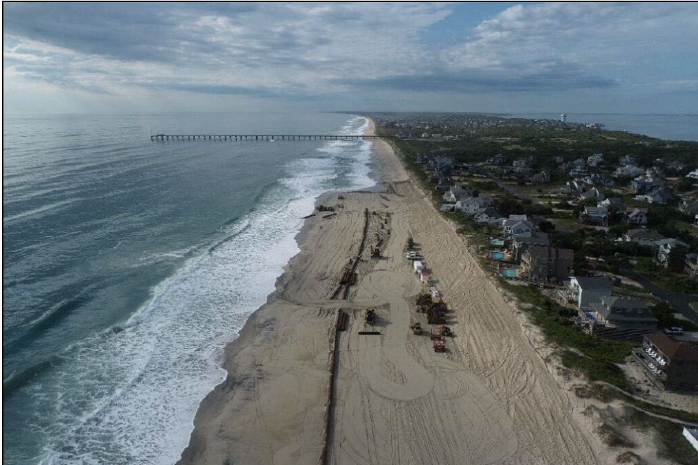
Figure 6. Duck, North Carolina, 2017 beach nourishment. USACE Field Research Facility research pier is visible at the top of the frame. (Image reproduced with permission from the Town of Duck and Coastal Planning and Engineering of North Carolina.)
