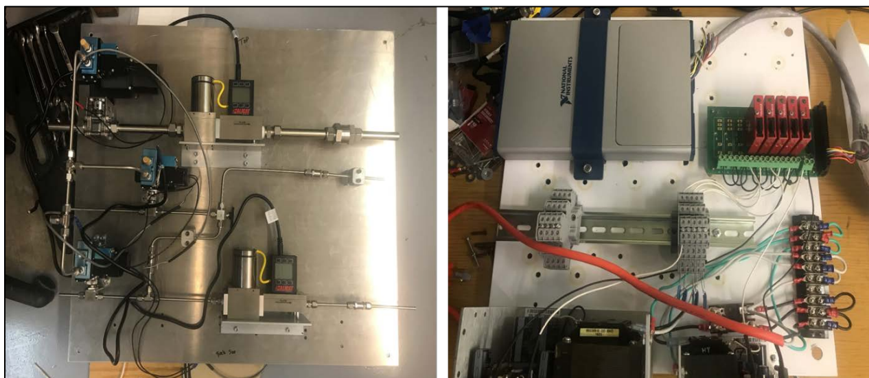
Figure 10: Plumbing panel for fuel, air, and purge gas (nitrogen) delivery (left) and the experiment control and data acquisition (DAQ) panel (right).
