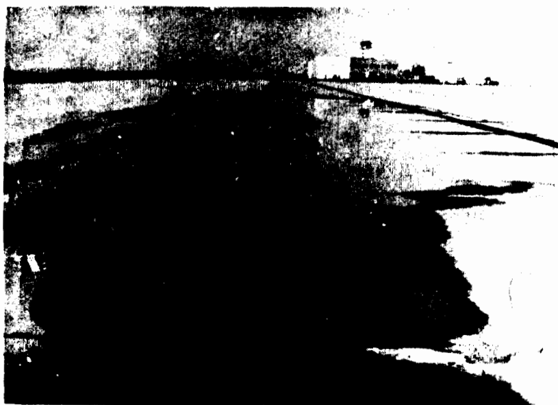
Figure B-3. Large "birdbath" in a taxiway leading to an Aircraft Parking Apron; large, wide areas such as this are often very difficult to drain because of limited initial cross slopes.
