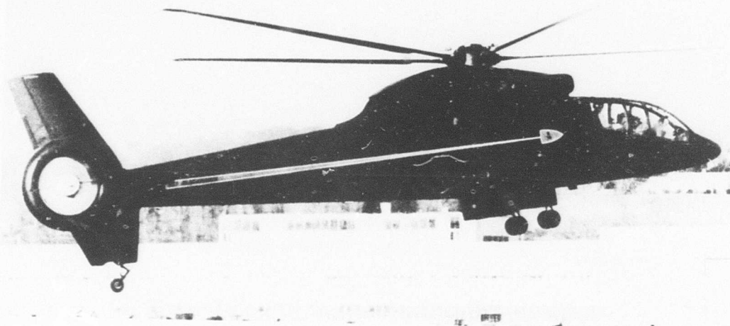
SIKORSKY S-67 MODIFIED FOR FAN-IN-FIN EVALUATION TESTING
