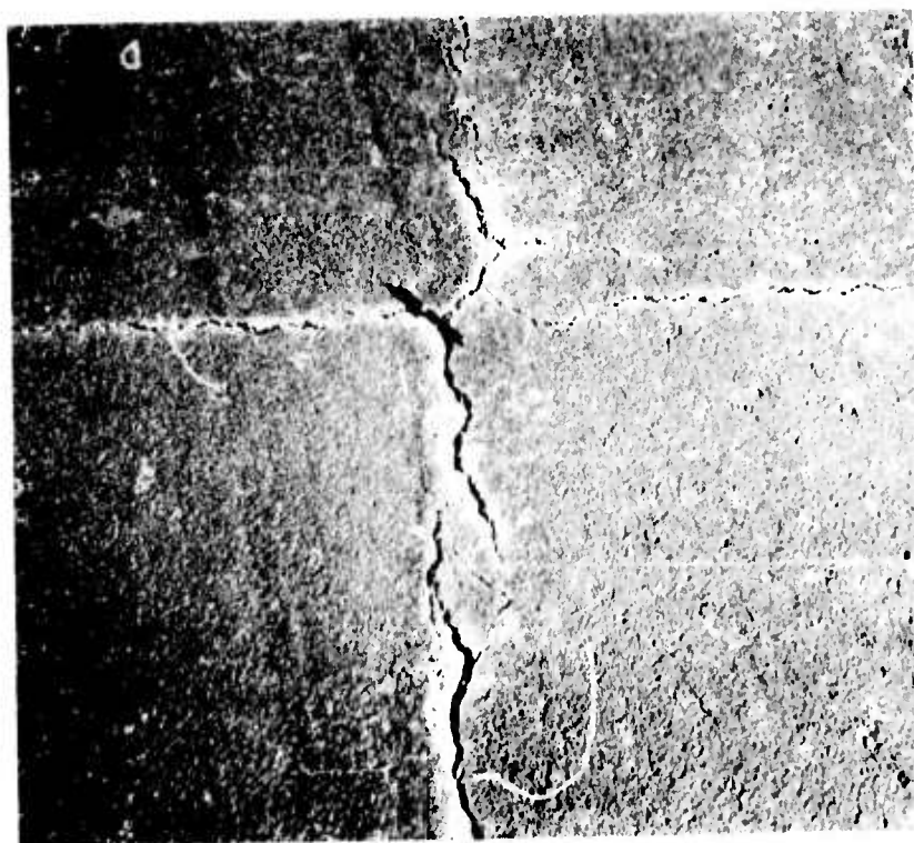
Photograph 5. Reflection cracking at slab intersections in apron area
