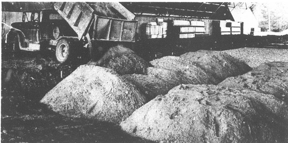
Fig. 3. End-dumping sand in item 4
