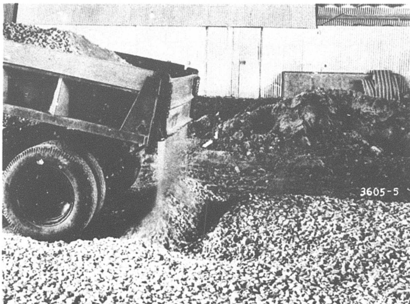
Fig. 2. End-dumping rock in item 3
