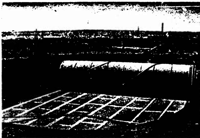
Fig. 7.12. Unrolling the rolled base of a 5,000 m 3 storage tank
