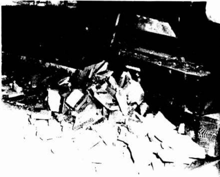
Debris Against Back Wall
