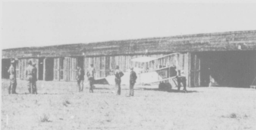
San Diego, Calif., became the site of the Army's first permanent aviation school. This is what the hangar line looked like in 1914, as war was breaking out in Europe.
