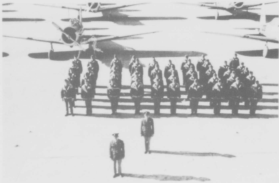
Cadets with Parachutes on Concrete Apron, 19 November 1942
