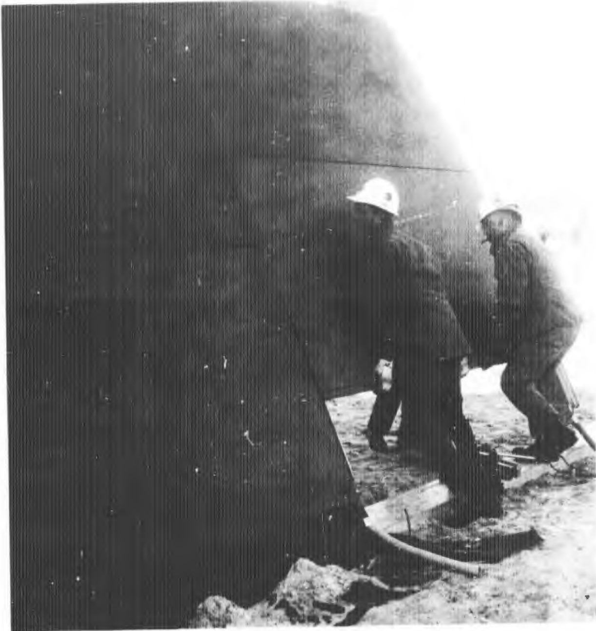
Figure 30 Installing Panel Manually
