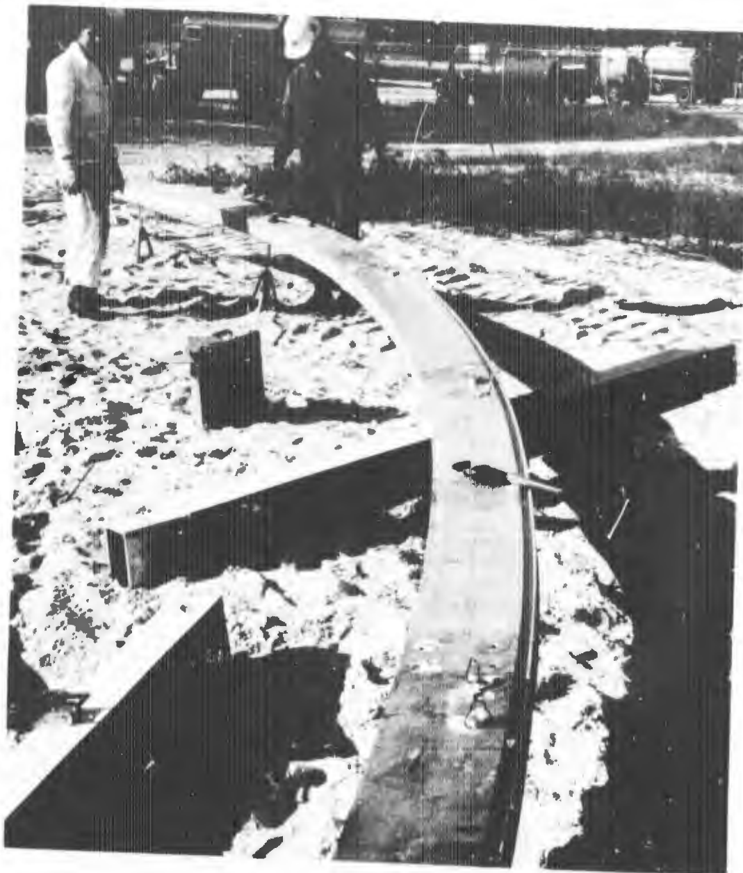
Figure 18 First Arch Beam Being Assembled
