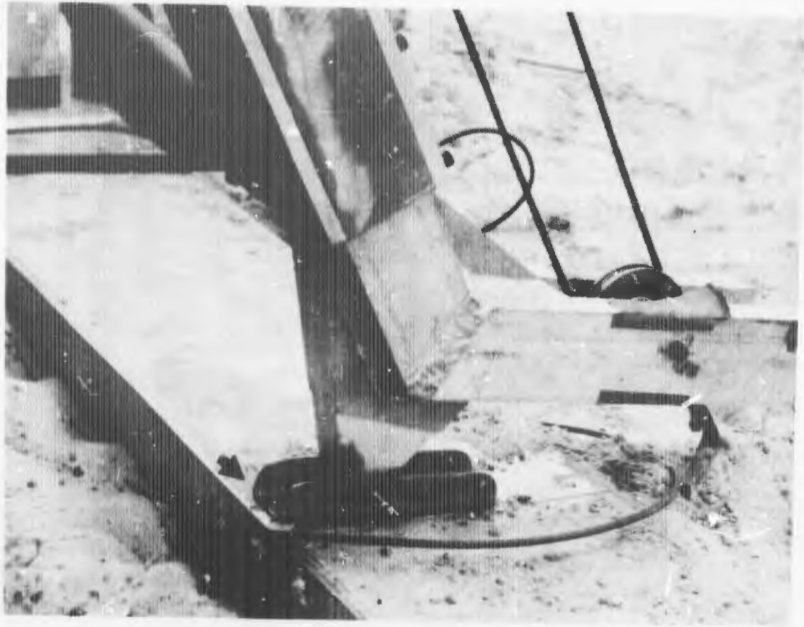
Figure 71 Base Attachment Raised During Panel Removal
