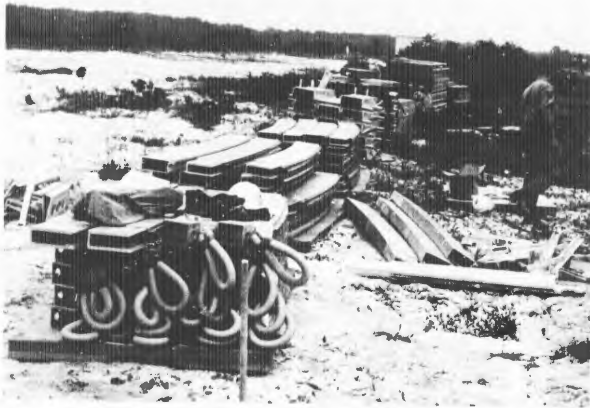
Figure 12 Palletted Shelter Components Prior to Erection
