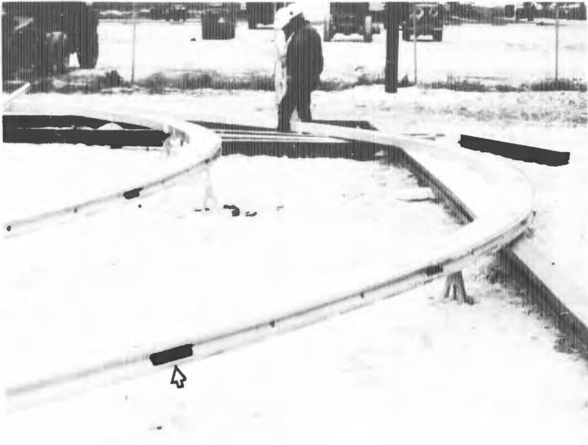
Figure 24 Arch Beam Assembly and Layout of Metal Door Frame Work
