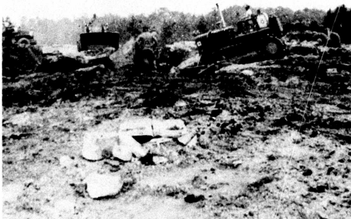
Figure 1.12 Pushing debris into crater.
