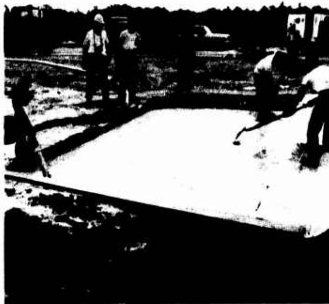
Figure 5.46 Placement of neat cement slurry cap.
