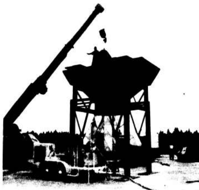
Figure 5.31 Gravity-feed cement storage hopper.
