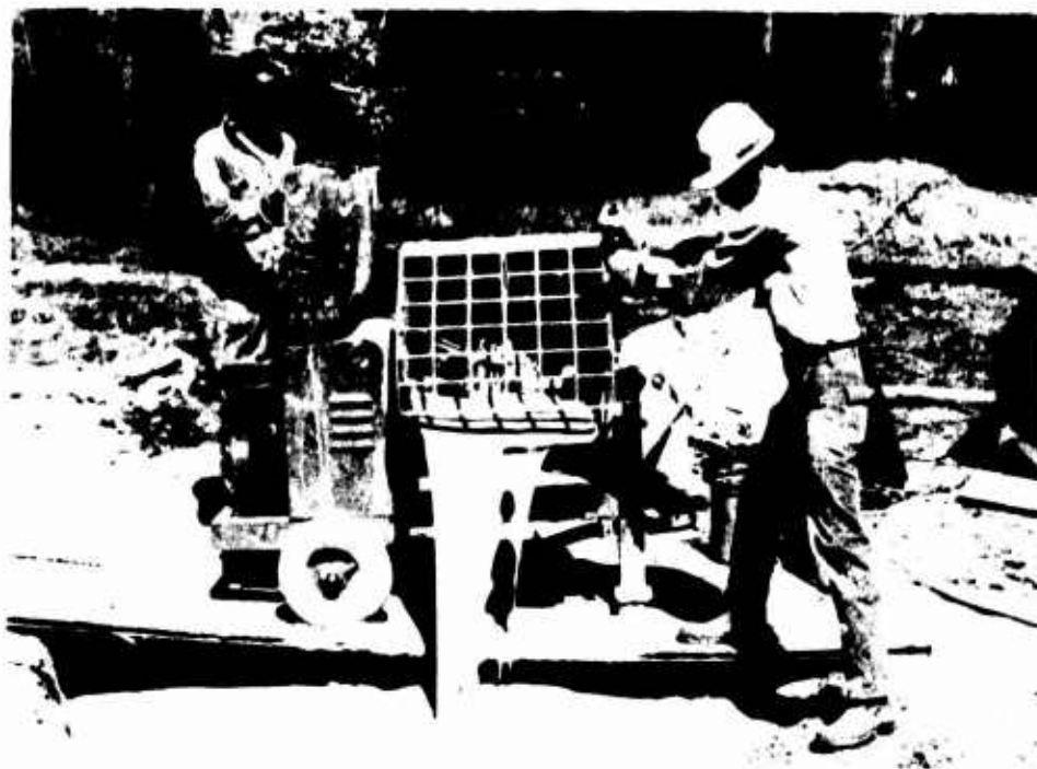
Figure 5.6 Placement of the 85-pcf cellular concrete.
