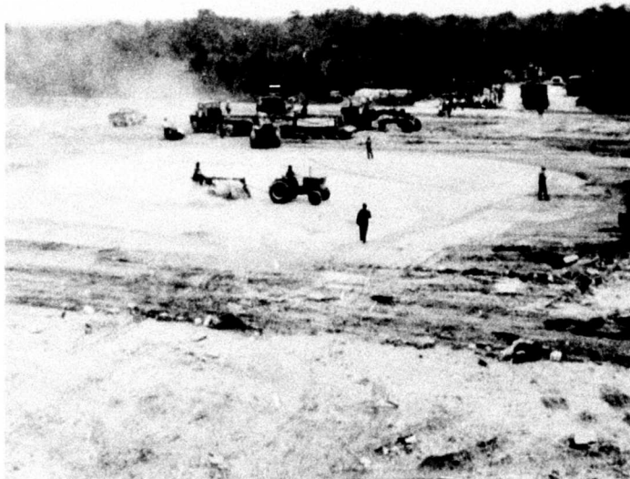
Figure 1.11 Sweeping adjacent area for mat assembly.
