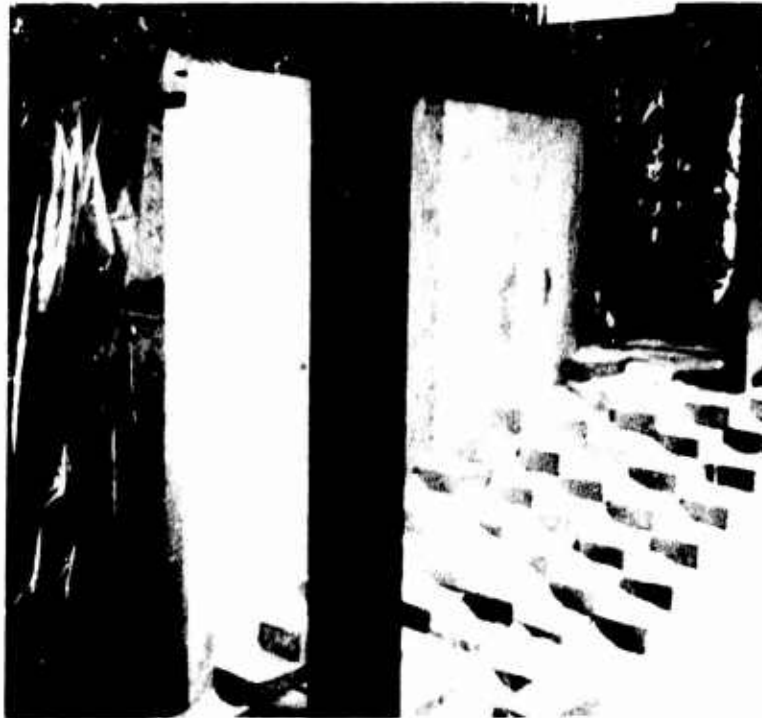
Figure 3. Early stage of constructing shield around tank. Note courses of stacked blocks with boric acid placed to fill joints. Plywood in center holds a 4-in.-thick vertical wall of boric acid
