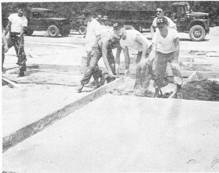
Figure 119. Screed Team Working Center Lane, Test 2-1
