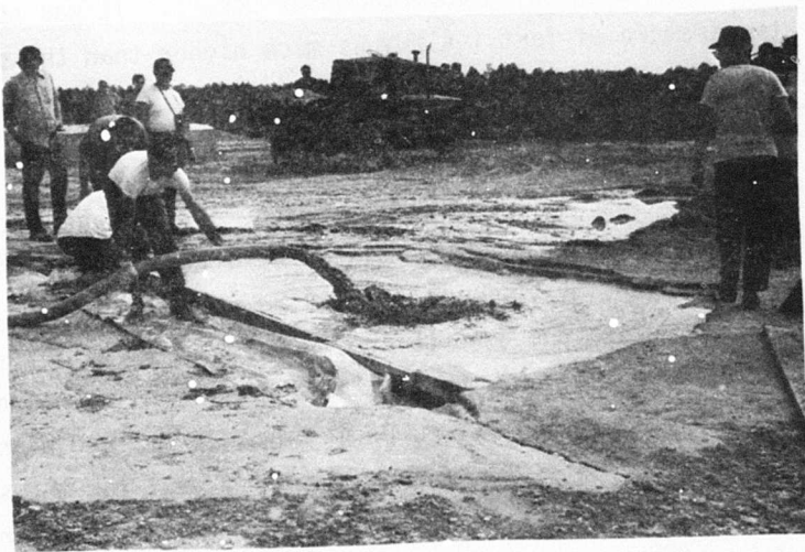
Figure 109. Reg-set Slurry Cap being Pumped on Crater 1-4 NW
