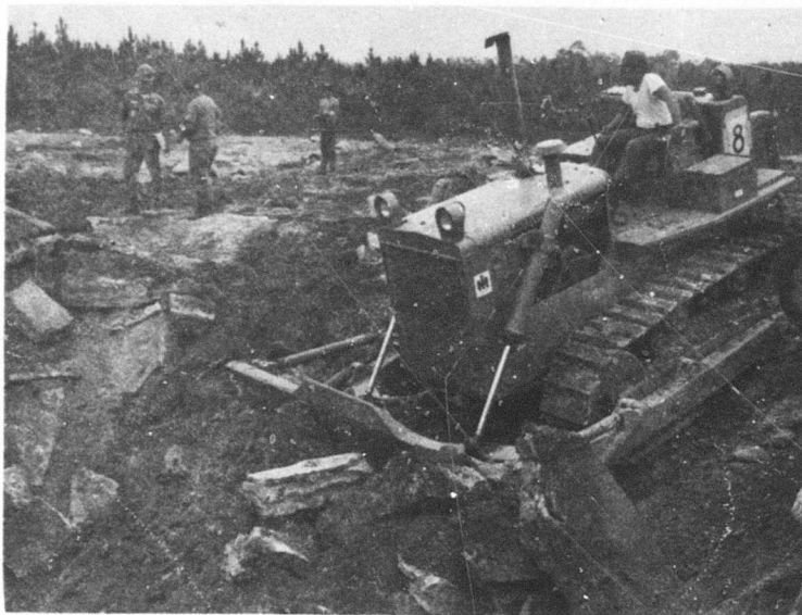
Figure 13. Test 1-1, TD 20 Full Tracked Dozer Pushing Large Debris Directly into Crater
