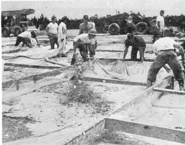
Figure 82. Test 2-1, Formwork being Filled with Reg-Set Cement Slurry
