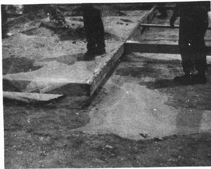
Figure 121. Reg-set Running Beneath Polyethylene Form Liner and Out of Formwork, Test 2-1
