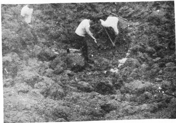
A. Preparing Grade for Block Loading
