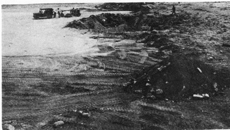
Figure 46A. Test 1-2, Upheaved Pavement Cleared of Debris on the Left
