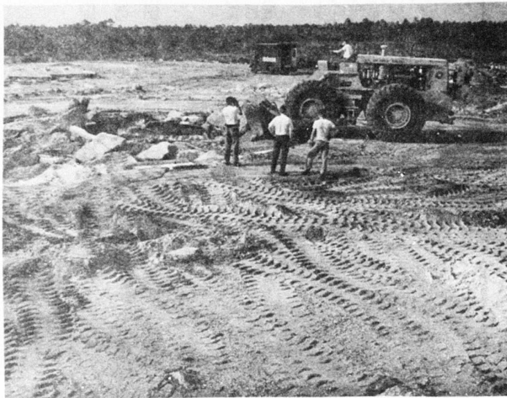
Figure 59. Test 1-3, 280 RT Completing Initial Encirclement of Crater
