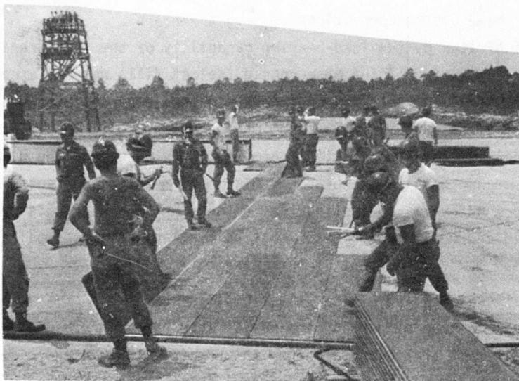
Figure 20. Test 1-1, AM-2 Airfield Patch Being Assembled
