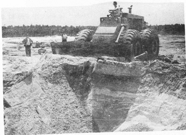
Figure 51. 280 RT as Used in Test 1-3, Pushing Debris Directly into Crater
