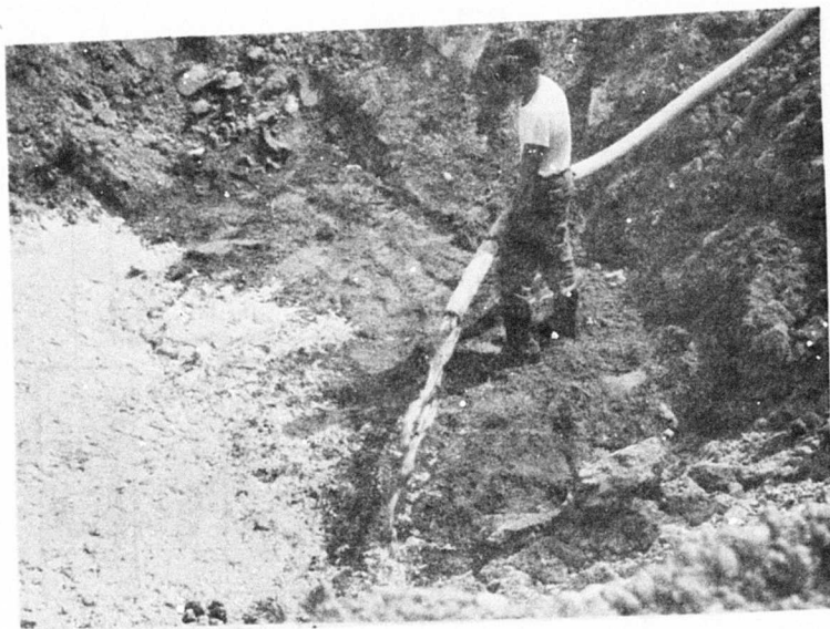
A. Placing Slurry Floor
