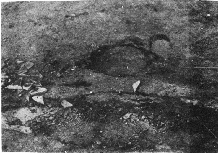
Figure 90. Test 2-1, Punching Failure, Middle, and Concentric Crack, Lower
