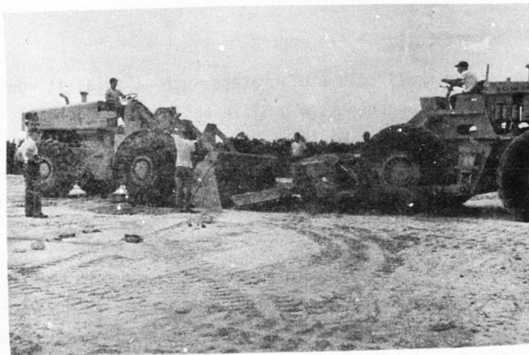
Figure 69. Test 1-4 NW, 280 RT and AC 745 Working on Crater Repair
