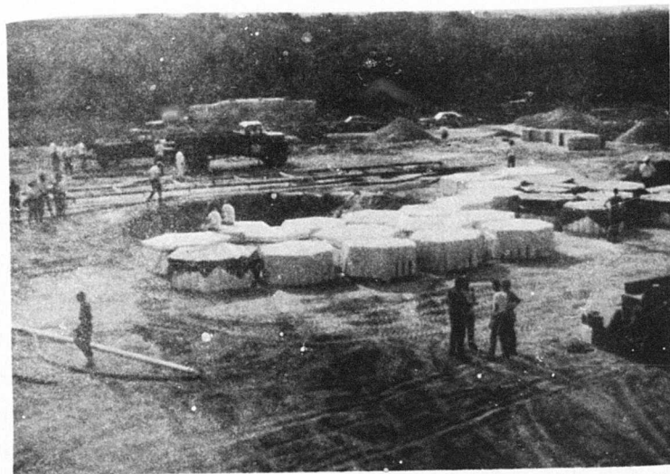
Figure 81. Test 2-1, Modules and Formwork at Site Prior to Test
