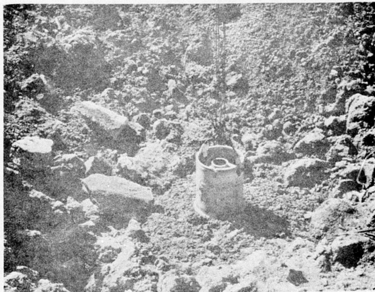
Figure 34A. Test 1-2, Backfilling Procedure Utilizing Cylinder to Form Column for Sensors
