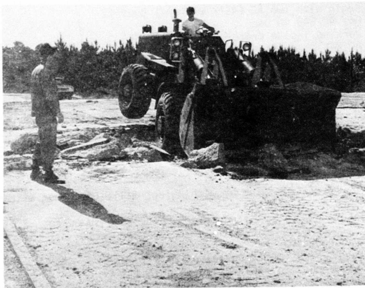
Figure 65. Test 1-4 NE, AC 645 Removing Upheaved Pavement from Inside Crater
