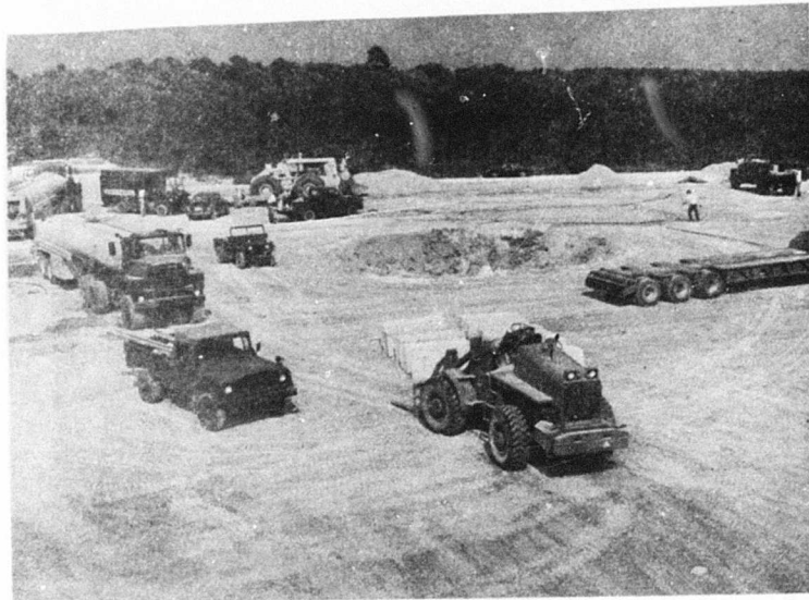
Figure 80. Test 2-1, Crater Following Area and Lip Cleanup and Internal Shaping
