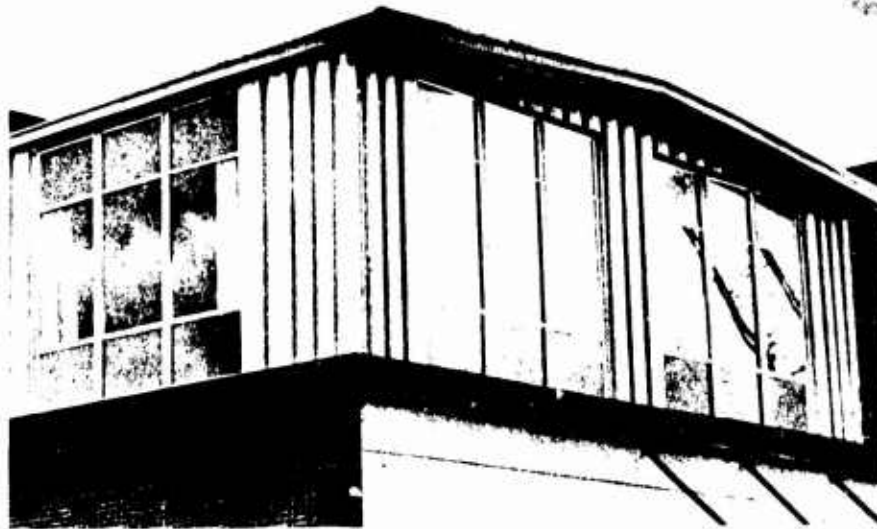
Figure 7. Northwest corner of cafeteria addition (metal building). Black arrows point to insulated porcelain-enamel panels. White arrow points to location of heat leak at roof-wall joint of metal building.
