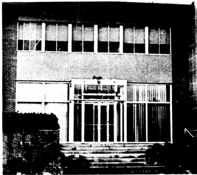
Figure 3. Main entrance of USACRREL building. Black horizontal arrows point to south-facing slate wall. White horizontal arrows point to east-facing slate wall. Each of six vertical arrows points to window with an installed storm sash.
