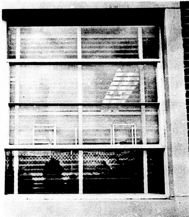
Figure 2. Typical window at USACRREL.
