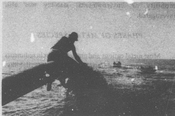
Photo 2. Sampling slurry from pipeline discharge
