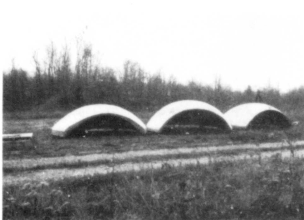
Figure 8. View of three domes tested.
