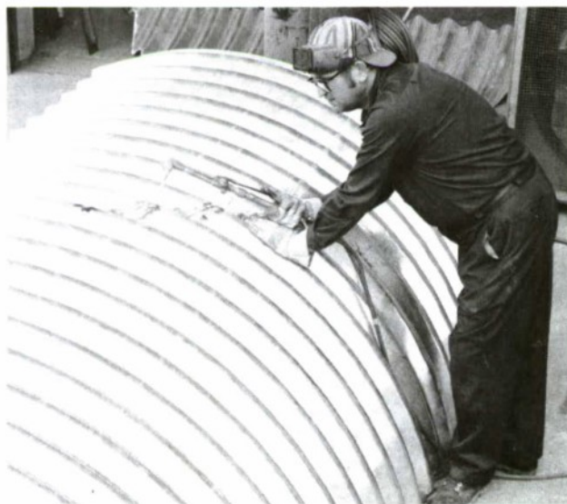
c. Cutting out the quarter-section
