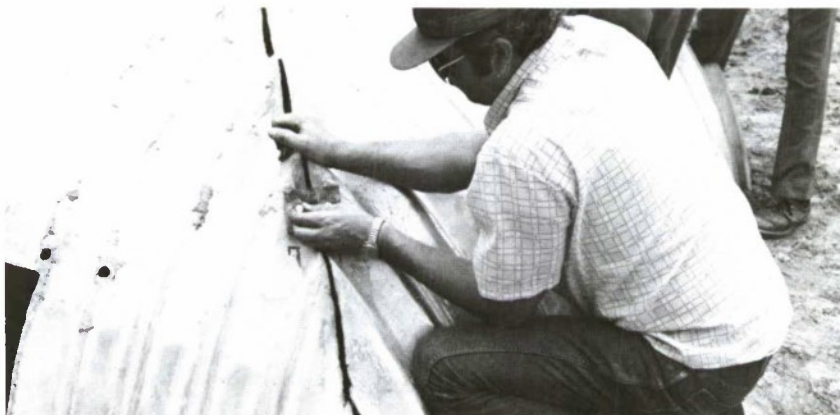
f. Attaching two adjacent quarter-sections with steel plates and bolts
