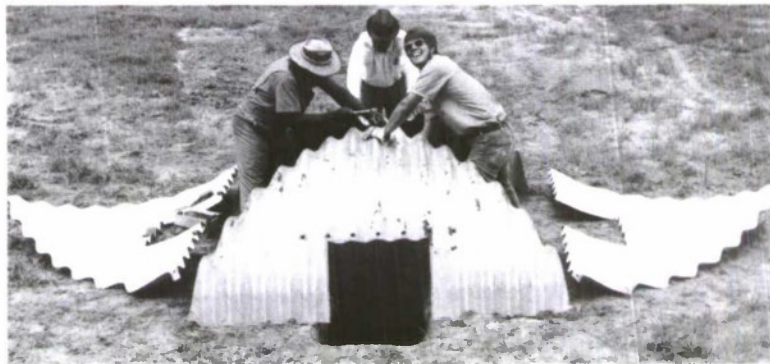
c. Attaching two quarter-sections of MICS
