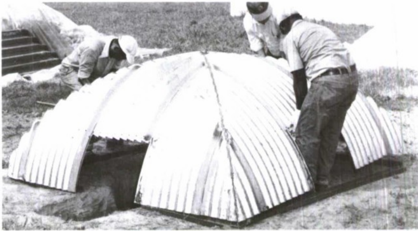
b. Three-man workcrew placing MICS
