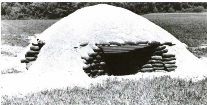
l. Completed bunker
