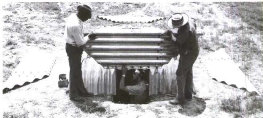
h. Attachment of an aperture beam
