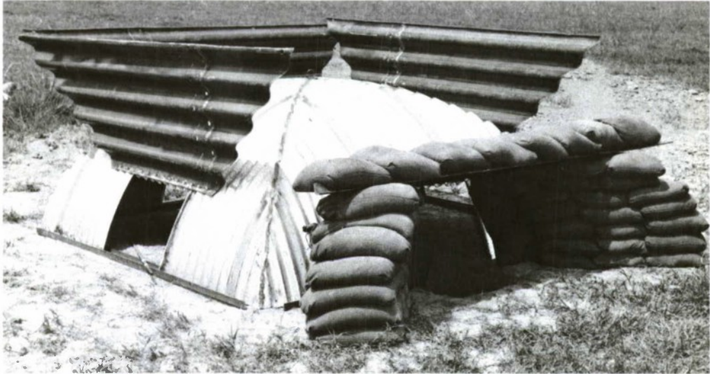
d. Sandbags placed over and under one aperture beam
