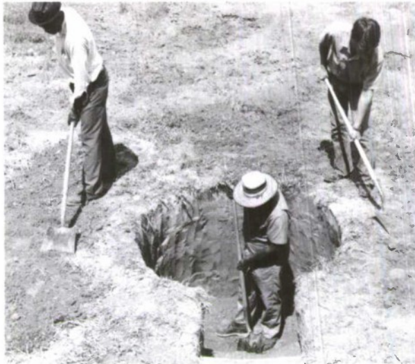
a. Excavation of fighting hole
