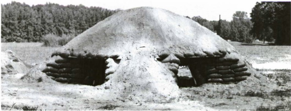
e. Sand cover placed over structure
