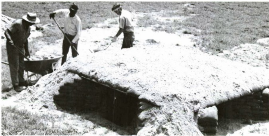
k. Placement of sand cover
