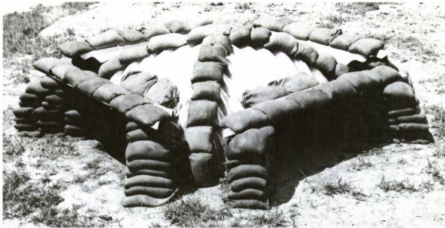
j. Completed assembly of prefabricated components with sandbags
