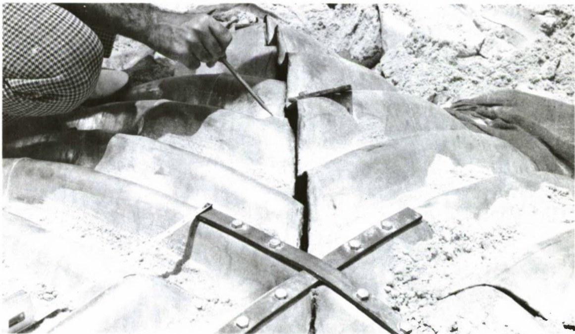
d. Deformed metal around a bolt hole
