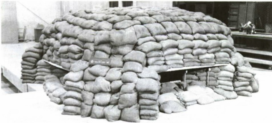
g. Seven layers of sandbags
