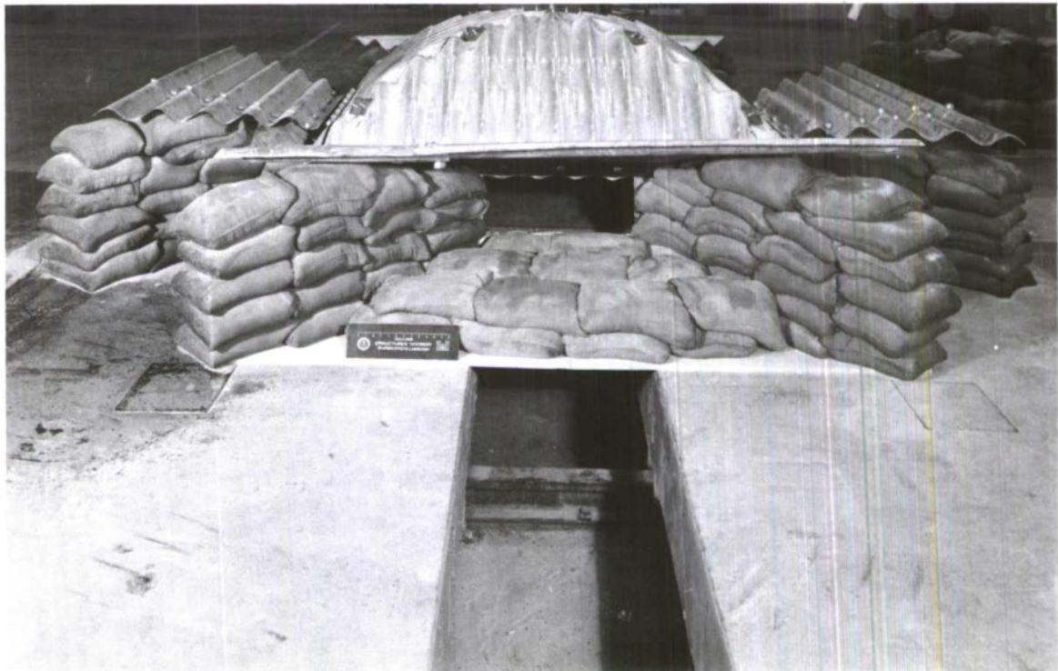
b. Test structure showing the 2-ft-wide entrance
