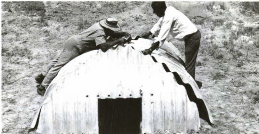
d. Attachment of last two quarter-sections at crown of MICS
