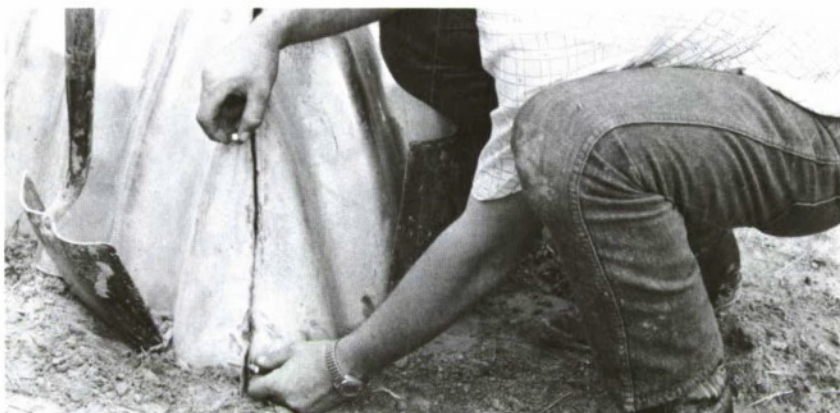
e. Attaching two adjacent quarter-sections of MICS at bottom
