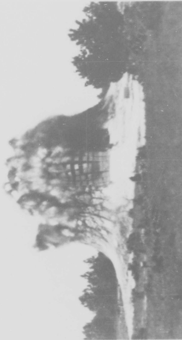
Figure 2. Early stage of venting of 12 MS event detonation, showing separation and lofting of runway pavement over crater area and initial upheaval of runway beyond crater edge.
