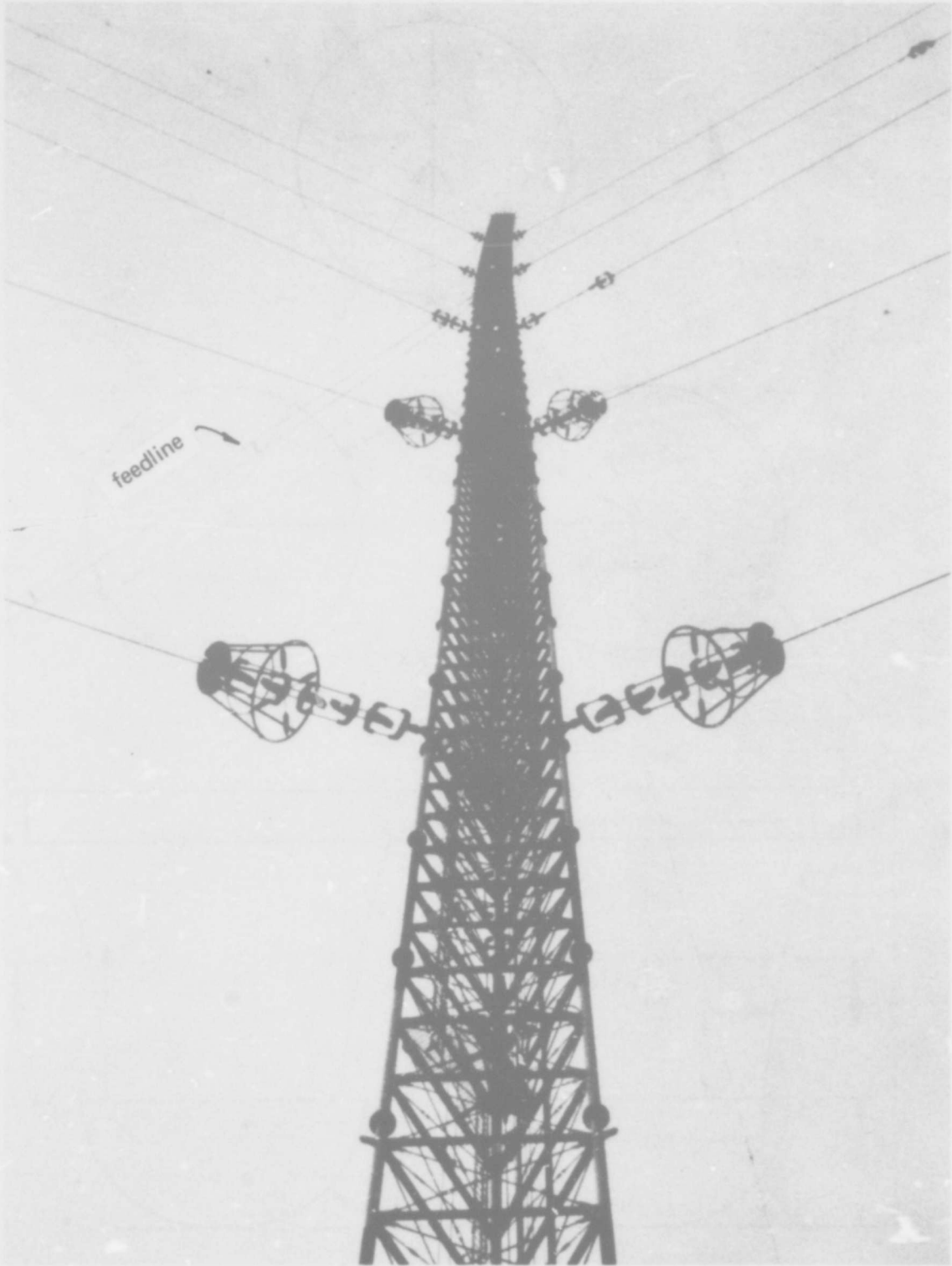
Figure 5. Eccentric displacement at fourth guy level from feedline pull.
