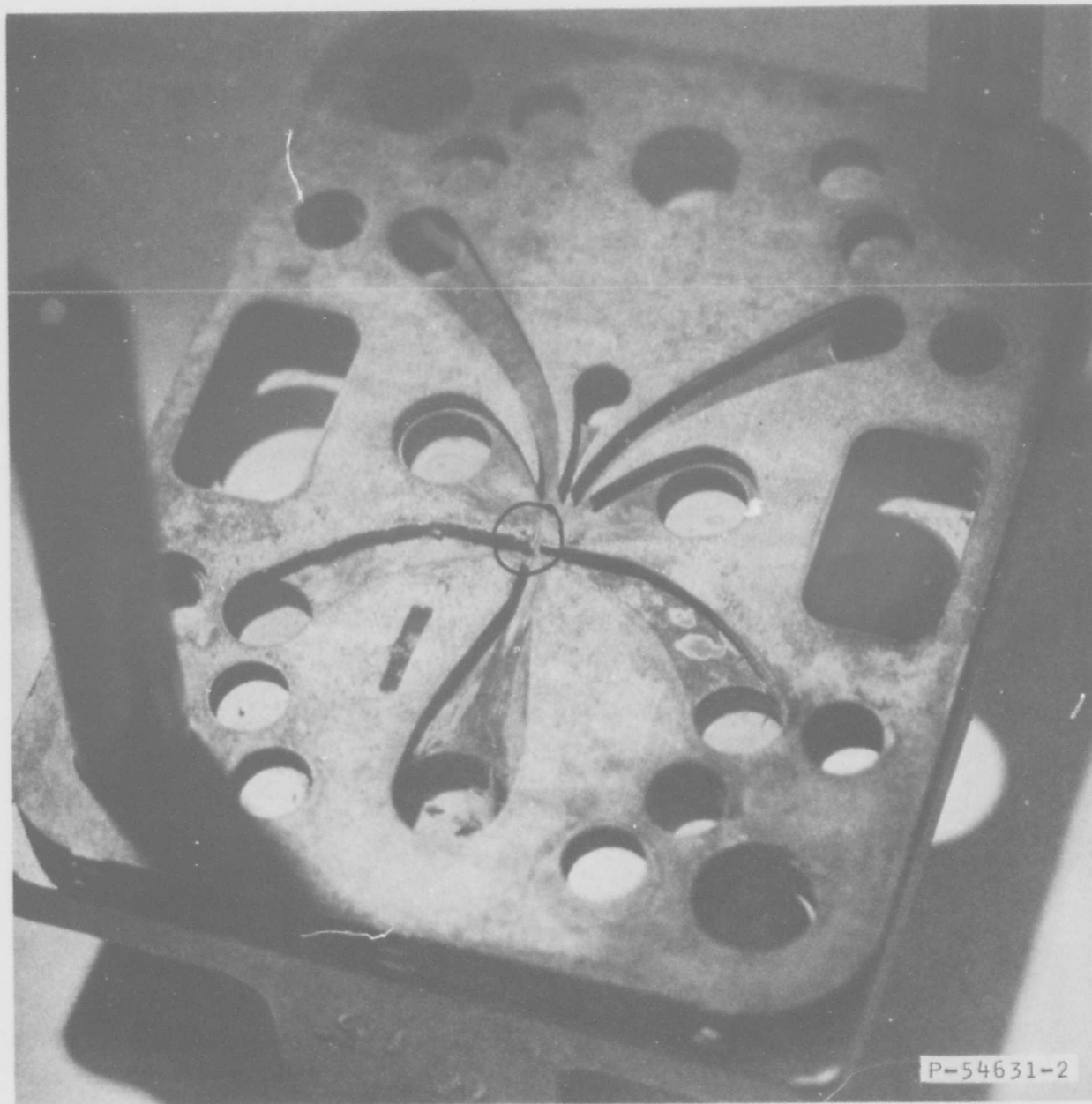
FIGURE 33 UNFILTERED BLEED AIR PARTIAL BLOCKING OF THIRD STAGE VENT RUN 2, STATION 1, LAMINATION 27
