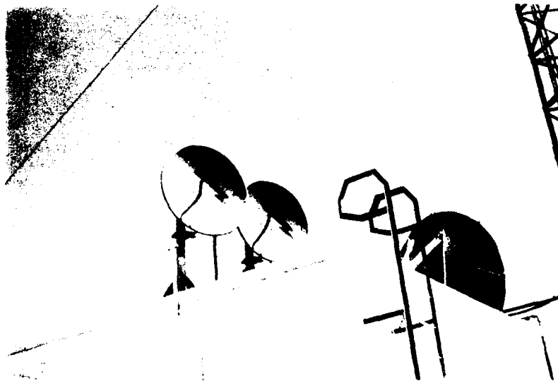
Figure 3. Receive antennas at Boone site.
