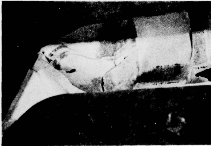
Figure 16. Additional Polystyrene Damage
