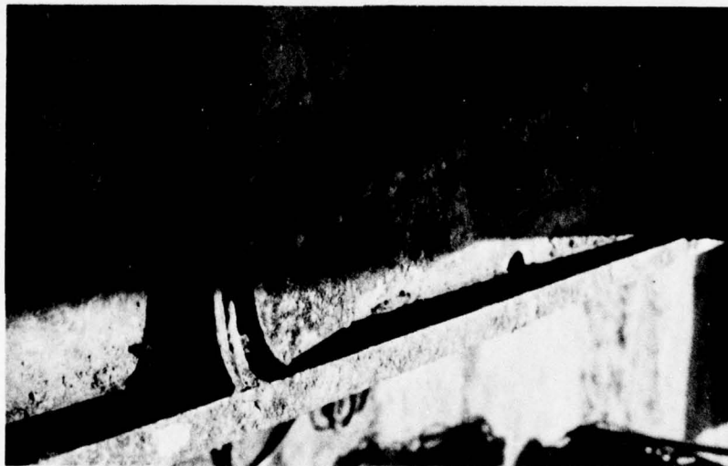
Figure A3. Typical rear support bar failure at both ends; lower end shown
