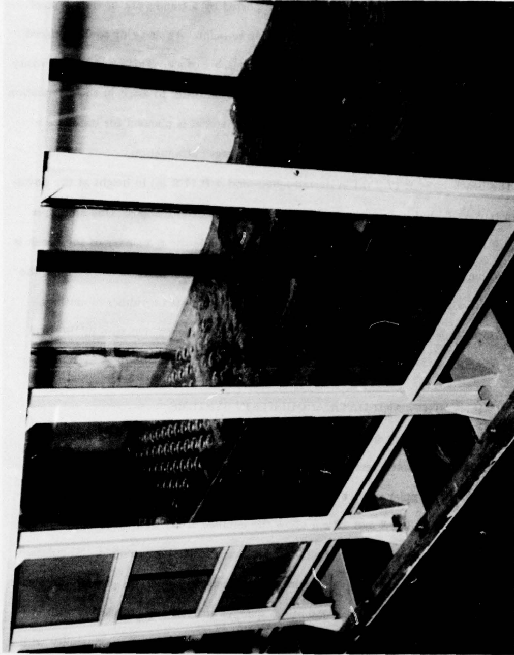
Fig. 5—The beach assembly installed in the channel
