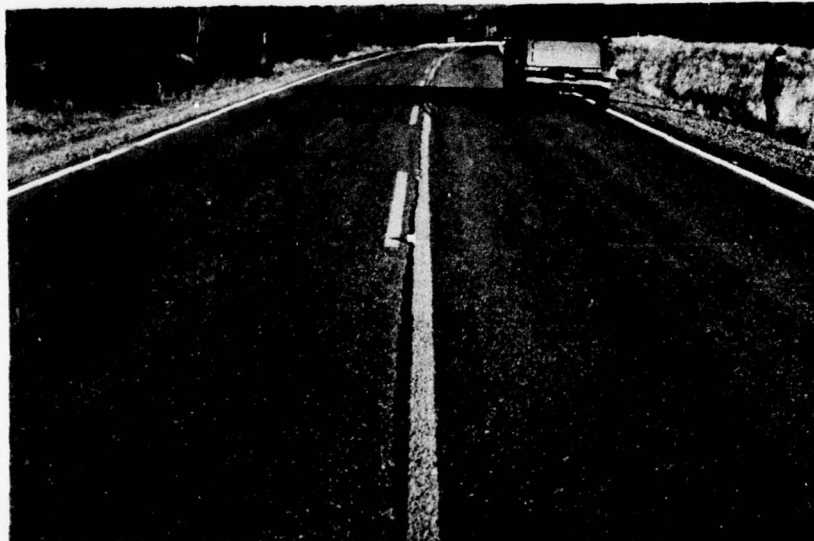
Figure 18. Longitudinal crack along center line.
