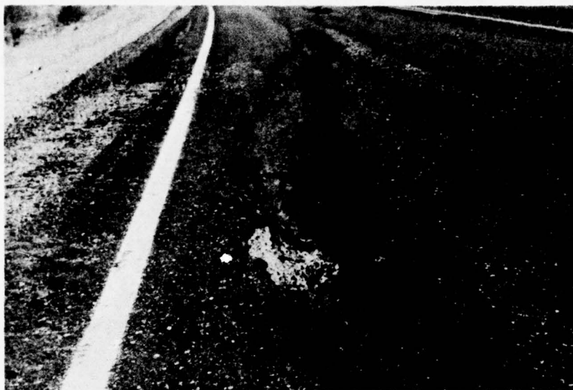
Figure 15. Pavement failure on Chena Hot Springs Road.
