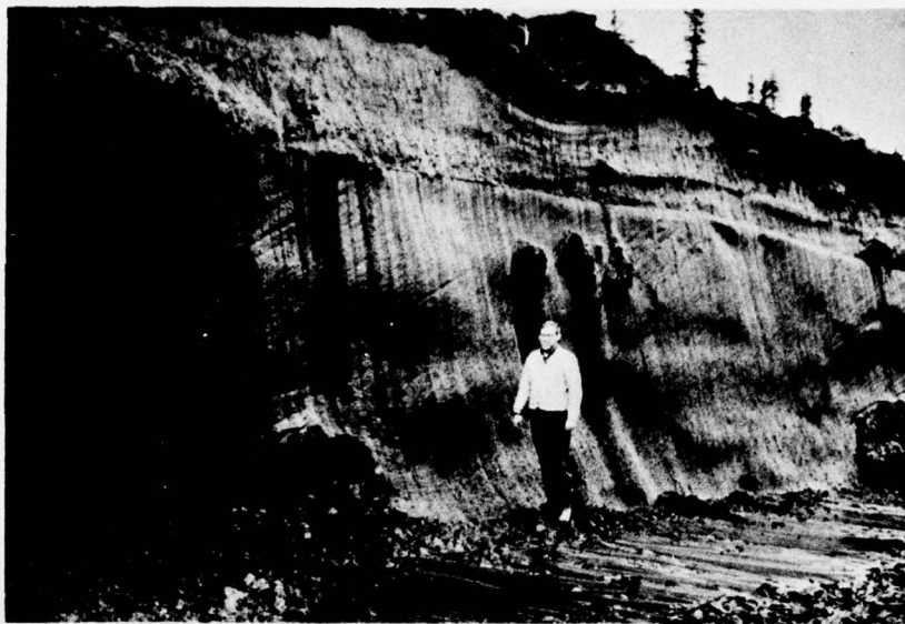
Figure 27. Vertical sidehill cut through ice at milepost 23.9 on TAPS road (from Smith and Berg 1973).
