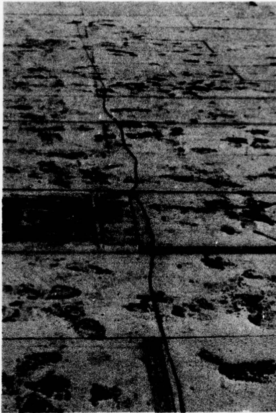
Figure 7. Polystyrene boards laid over a subbase prior to placement of fill.
