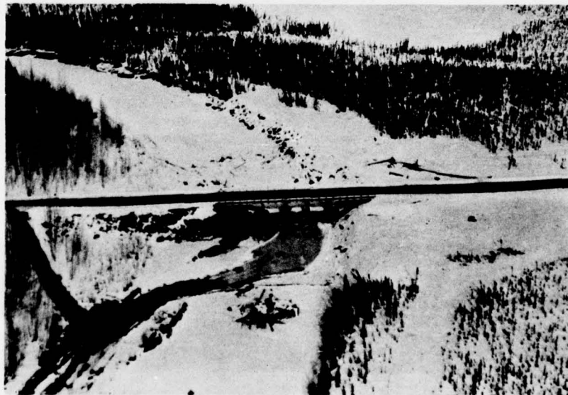
Figure 35. Hess Creek Bridge on TAPS road.
