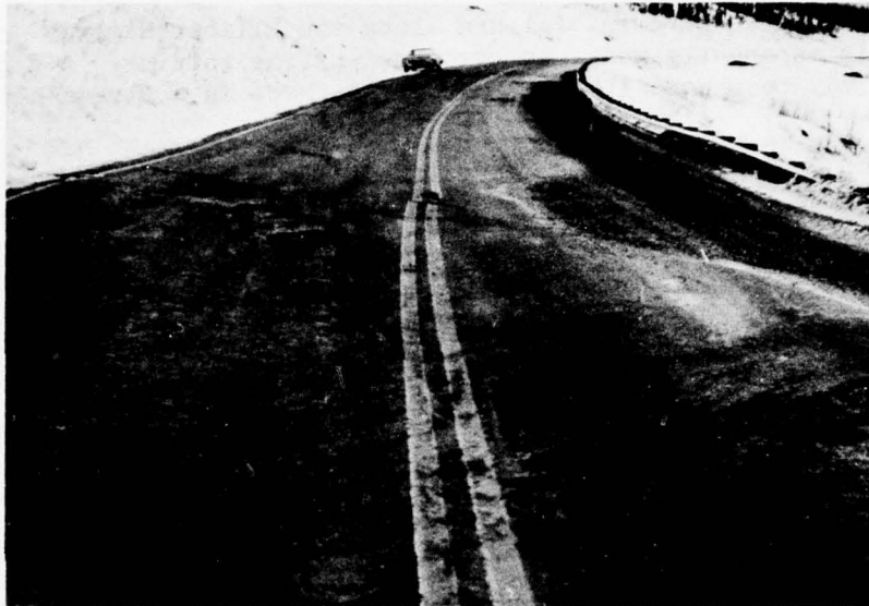
Figure 20. Creep on side hill on Steese Highway, mile 21.
