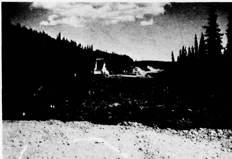
Figure 4. End dumping on Goldstream Road.
