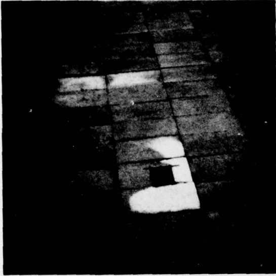
a. Stevens Hall roof drain.
