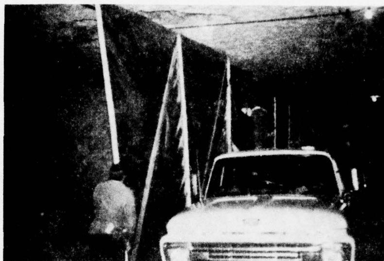
Figure 19. Installation of Panels to form Continuous Wall.
