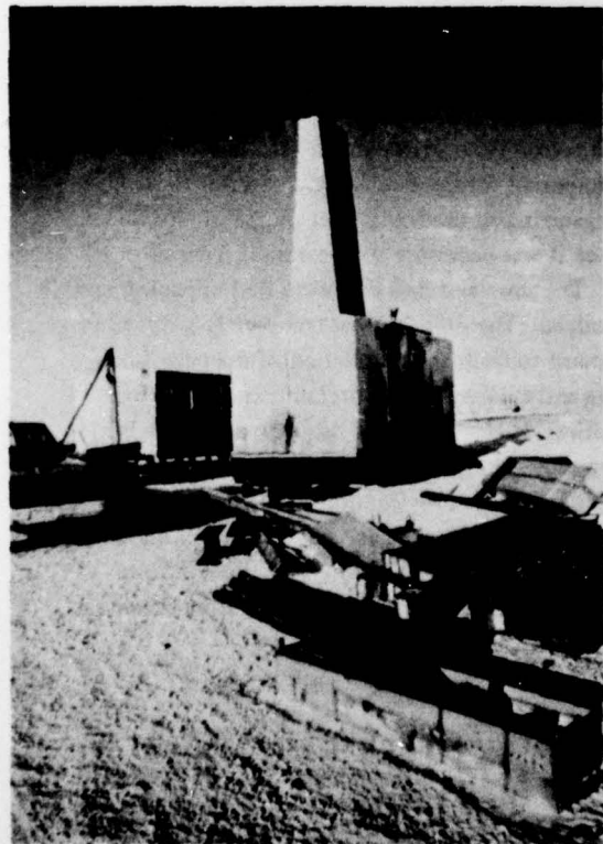
Figure 7. Drill sled being modified with new tower and drilling unit. In lower right the new Acker unit is being loaded on the Bombardier trailer for transfer onto the drill sled.
