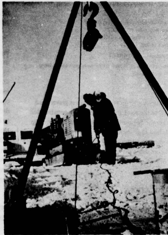
Figure 7. Drill sled being modified with new tower and drilling unit. In lower right the new Acker unit is being loaded on the Bombardier trailer for transfer onto the drill sled.
