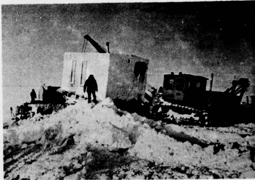
a. Snow ramp and tractor being used to load drill sled on the RD-85/RDT-45 tractor-trailer unit.
